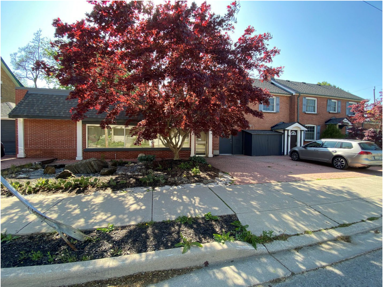
Image 3: Photograph looking west across Cathcart Street showing the full front façade of the existing house on the subject property including the one-storey commercial/storage portion to the south to be altered.
