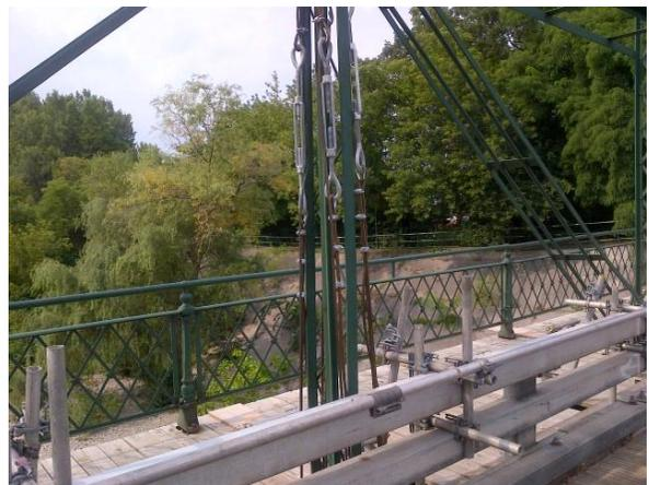
3. Temporary Repairs to Allow for the Reopening of the Bridge Sidewalk to Pedestrian Traffic
