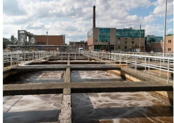
Greenway Wastewater Treatment Plant
