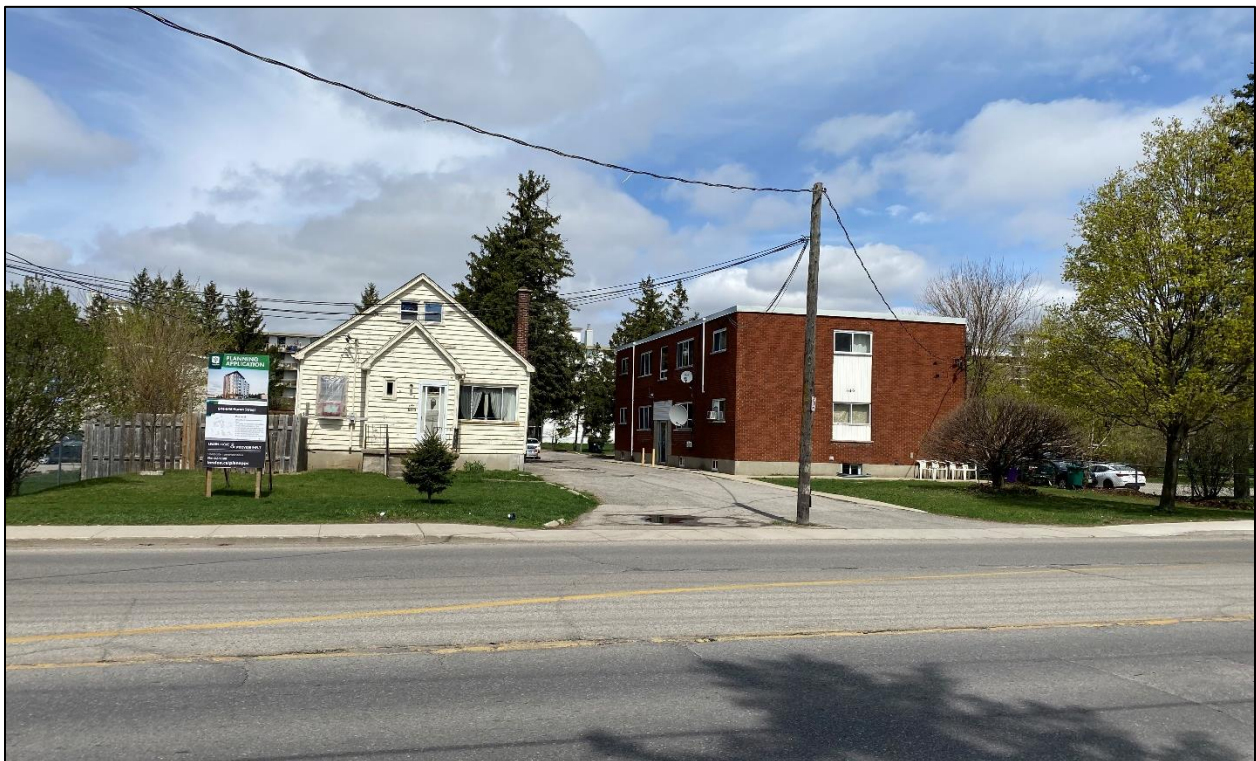
Figure 1: Photo of 644-646 Huron Street (view from Huron Street)
