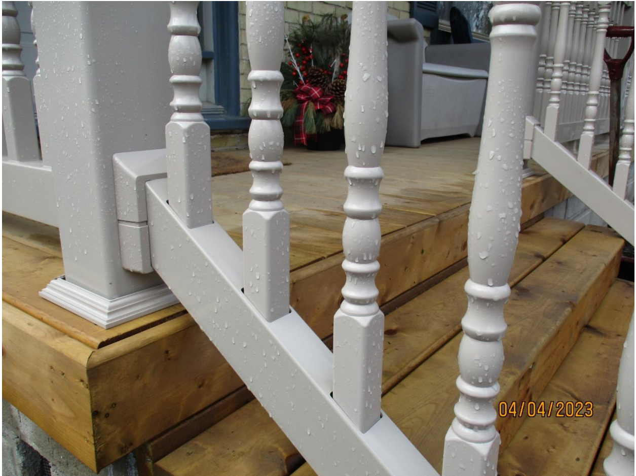
Image 7: Photograph showing detail of the vinyl (plastic) porch materials used for the replacement of the porch at 27 Bruce Street within the Wortley Village-Old South Heritage Conservation District.
