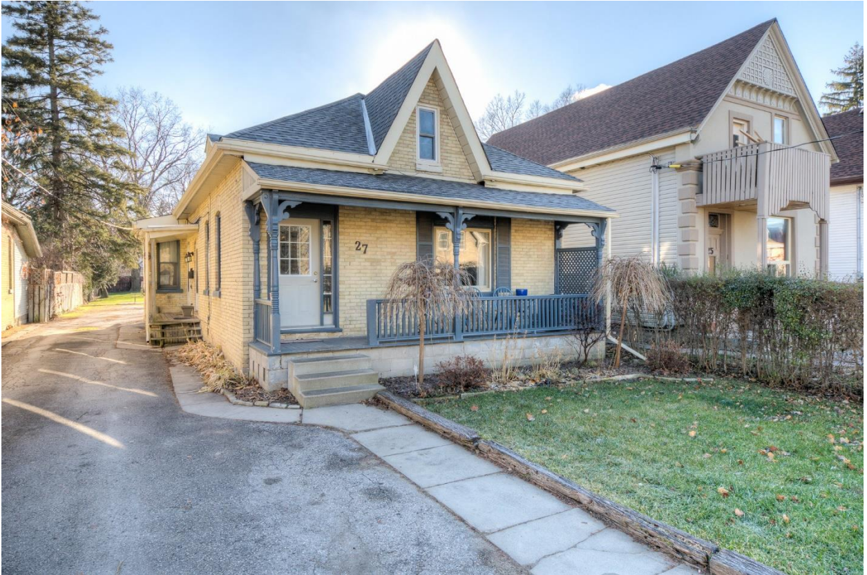
Image 1: Photograph submitted with the Heritage Alteration Permit application showing the previous porch prior removal without Heritage Alteration Permit or Building Permit approval. The porch posts and railings consisted of wood materials. The decorative brackets have also been removed.
