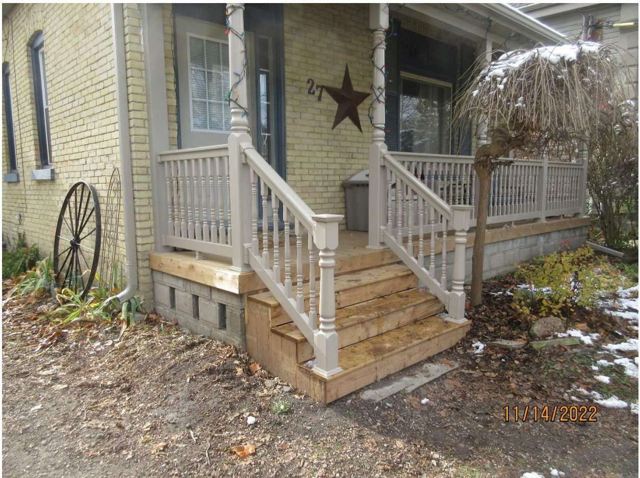
Image 4: Photograph showing detail of the vinyl (plastic) porch materials used for the replacement of the porch at 27 Bruce Street within the Wortley Village-Old South Heritage Conservation District.
