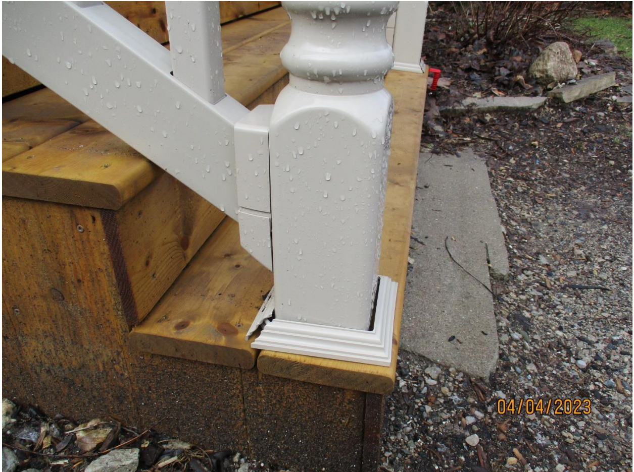
Image 5: Photograph showing detail of the vinyl (plastic) porch materials used for the replacement of the porch at 27 Bruce Street within the Wortley Village-Old South Heritage Conservation District.
