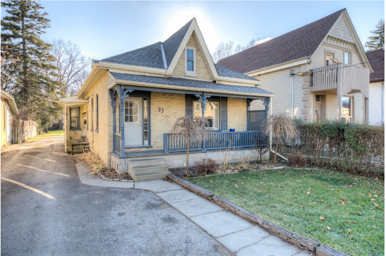
Image 1: Photograph submitted with the Heritage Alteration Permit application showing the previous porch prior removal without Heritage Alteration Permit or Building Permit approval. The porch posts and railings consisted of wood materials. The decorative brackets have also been removed.
