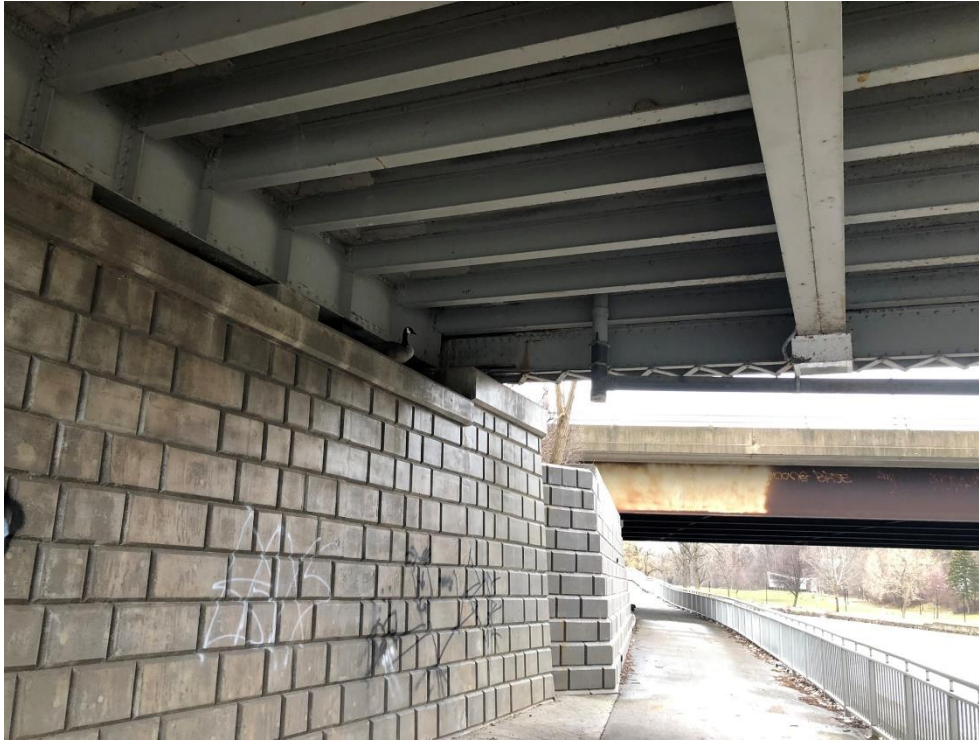
Photograph 28: West abutment with stone cladding (AECOM, 2022)
