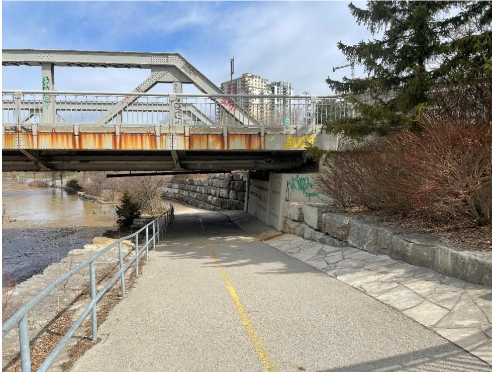
Photograph 20: View of the east end abutment and TVP below bridge (AECOM, April 2023)
