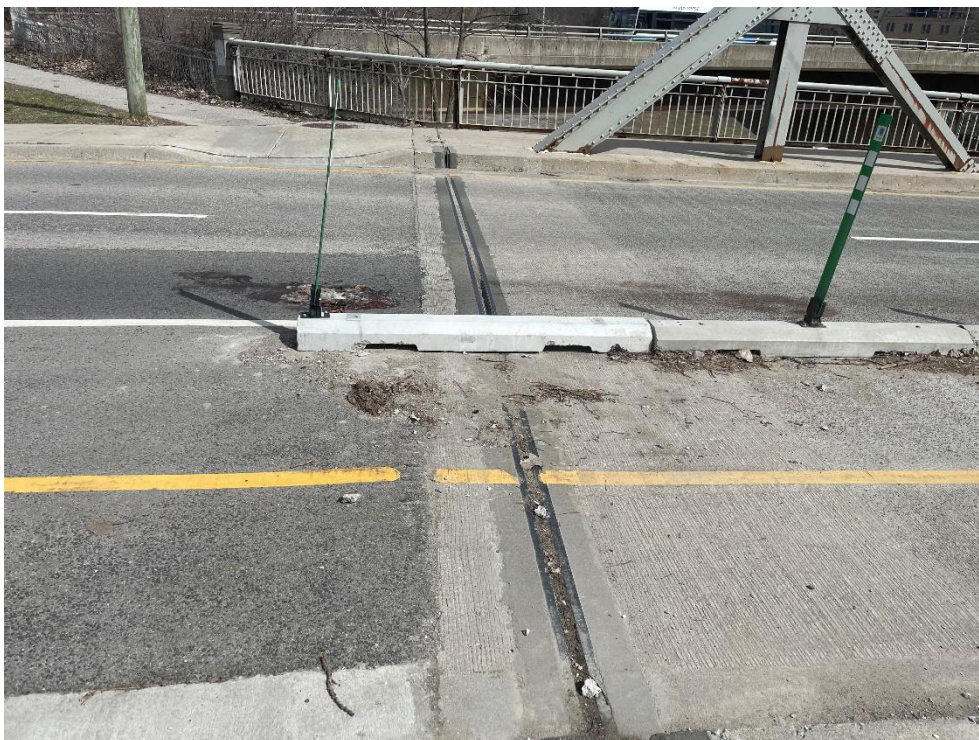
Photograph 11: West expansion joint over the abutment (AECOM, April 2023)
