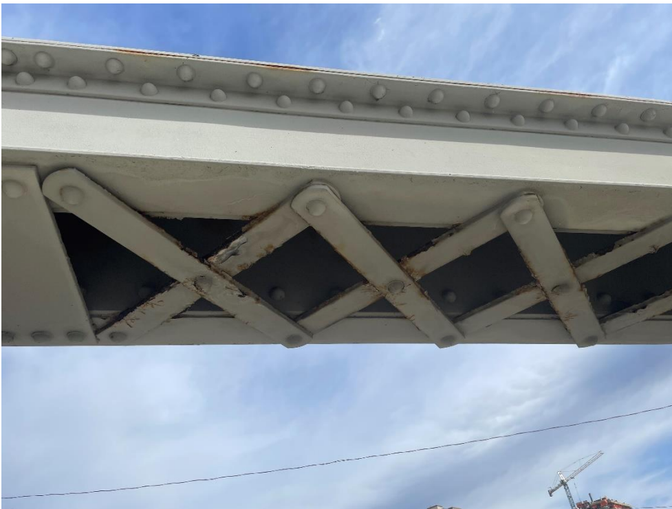
Photograph 13: Riveted lattice on the top chord (AECOM, April 2023)
