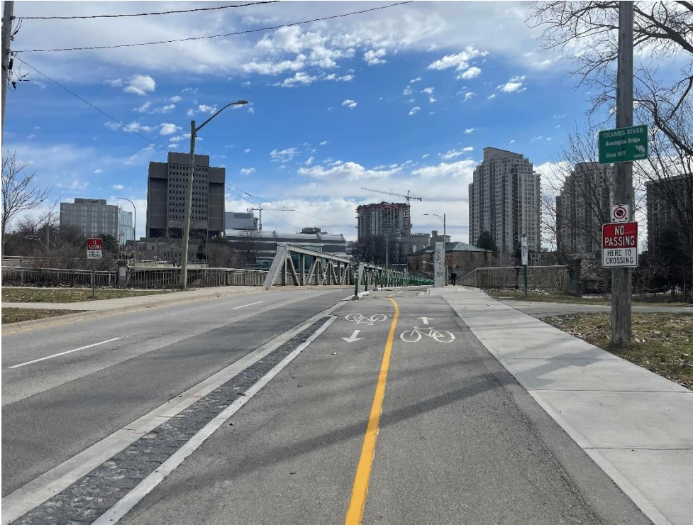
Photograph 2:View of bridge from Dundas Street, looking east (AECOM, April 2023)
