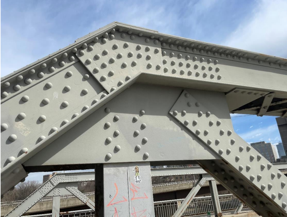
Photograph 12: Top chord connections, including steel gusset plates, as viewed from the south sidewalk (AECOM April 2023)
