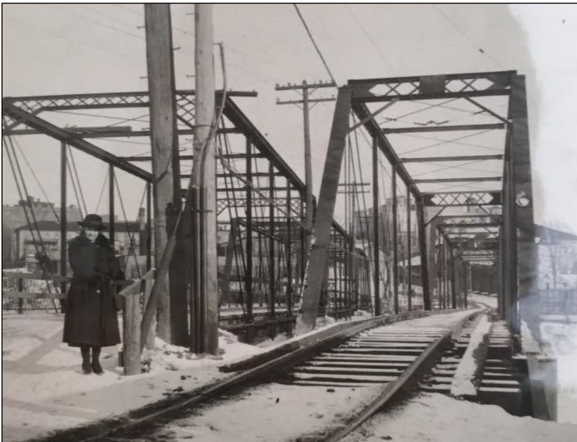
Image 4: View looking eastward toward Downtown London of the 1895 LSR bridge (on right) and the 1884 three-span Pratt truss bridge (on left), ca. 1923 (Western Archives. Western University. Regional Photograph Collection. RC60082) 3
