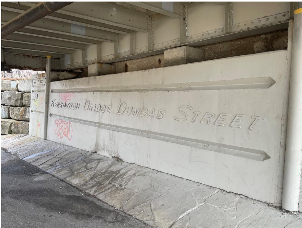
Photograph 21: Close-up of the east abutment (AECOM, 2021)
