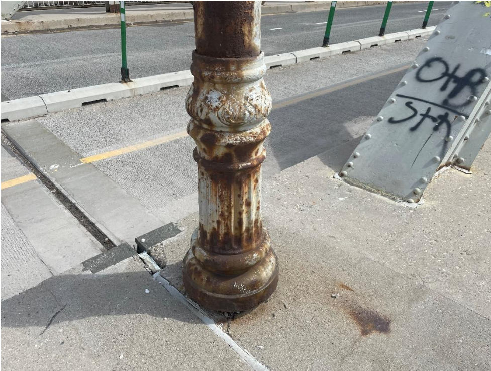
Photograph 16: Light post decorative sleeve on south side of bridge (AECOM April 2023)
