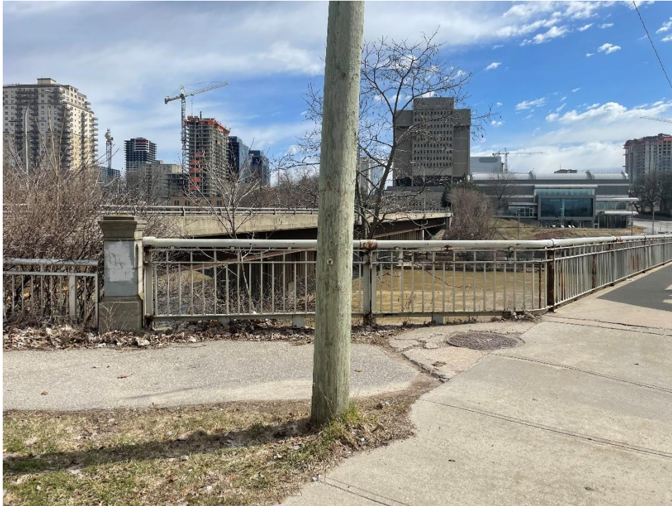
Photograph 10: Northwest concrete post and handrailing (AECOM April 2023)
