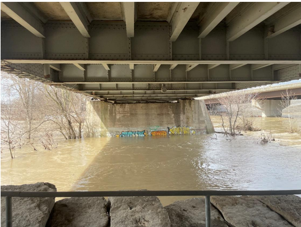
Photograph 23: View of the east pier from the underside of the east end of the bridge (AECOM, April 2023)
