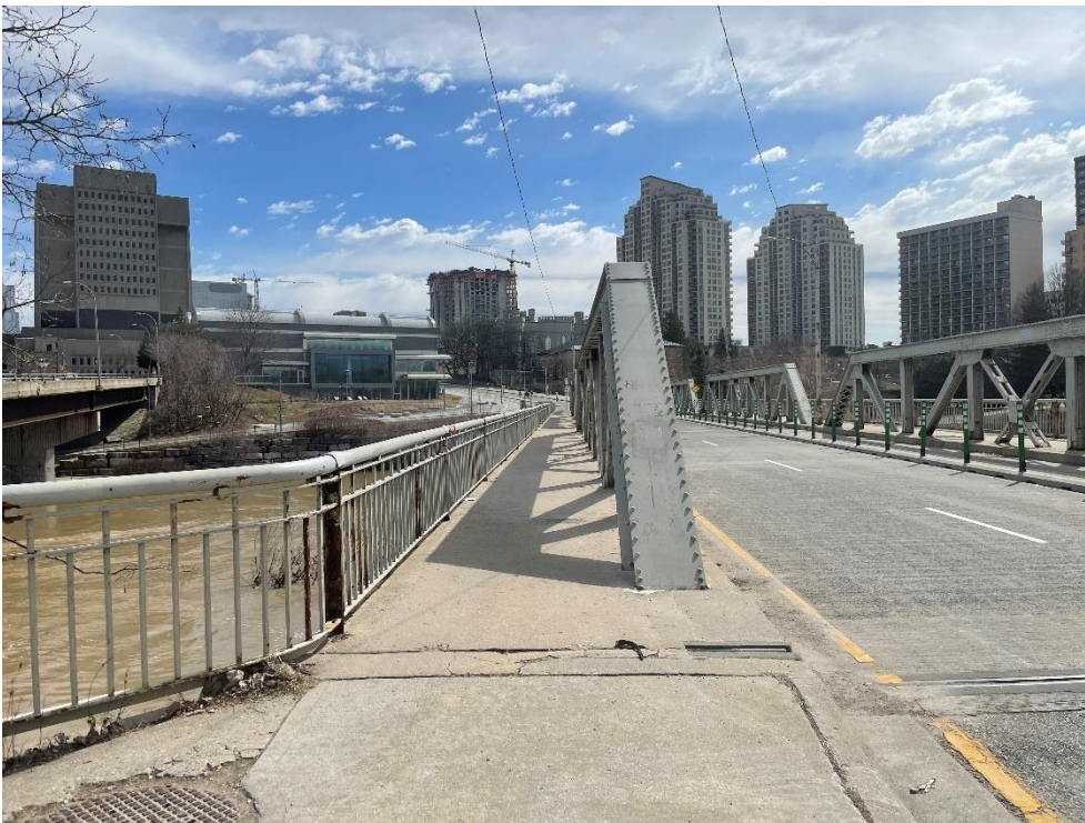
Photograph 5: Sidewalk portal view on north side, looking east (AECOM, April 2023)
