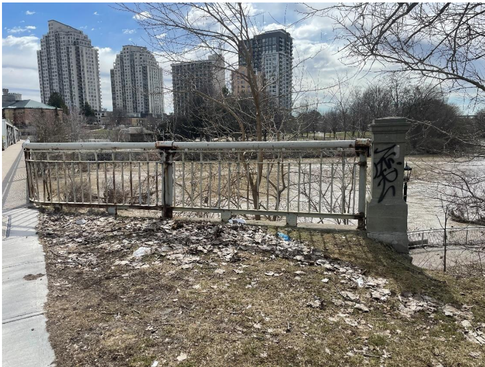
Photograph 9: Southwest concrete post and handrailing (AECOM, April 2023)
