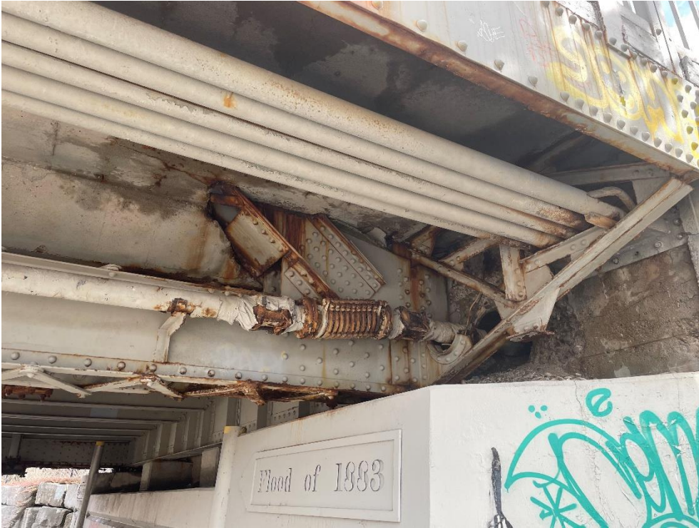
Photograph 22: View of underside of bridge at the east abutment with conduits (AECOM, April 2023)
