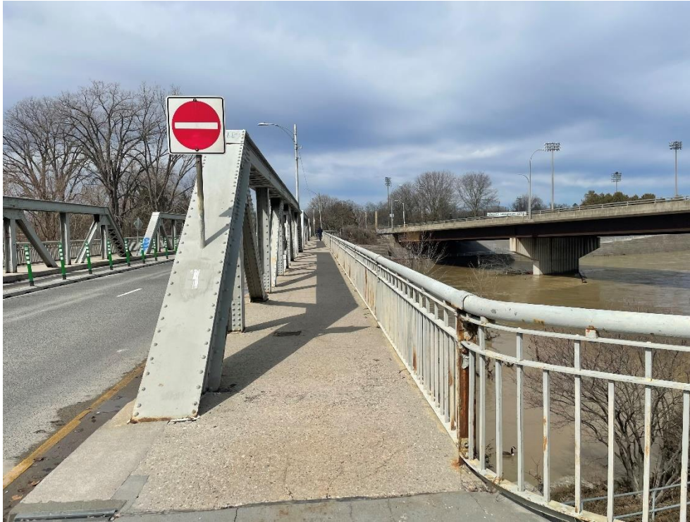
Photograph 8: Sidewalk portal view on north side, looking west (AECOM, April 2023)
