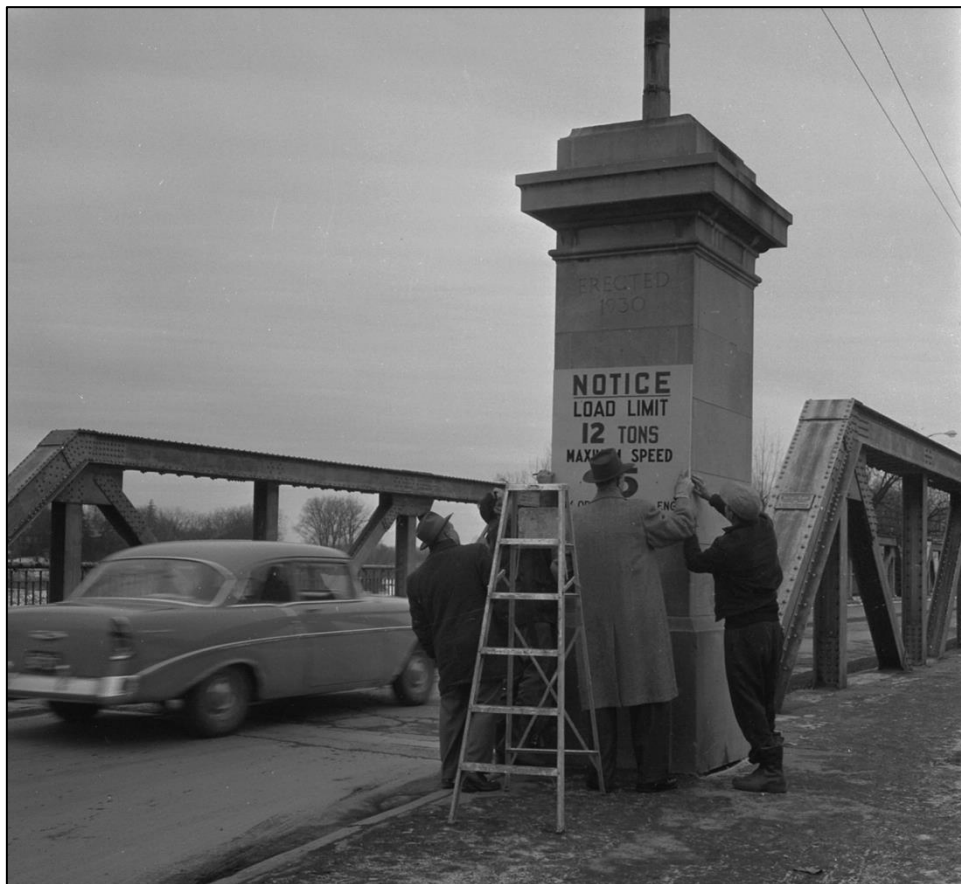
Image 5: Pillar with load limit and a date stone “Erected 1930” (Western University, London Free Press, January 9, 1960)
