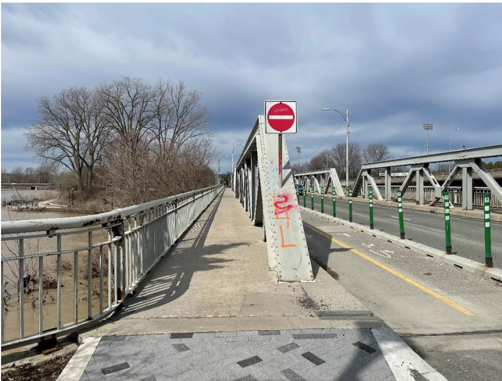
Photograph 7: Sidewalk portal view on south side, looking west (AECOM April 2023)
