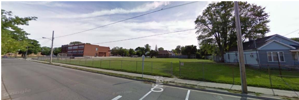
6 Street View of school the south west portion of the school building (1952 addition) from the bottom of the property / Source: Google Maps
