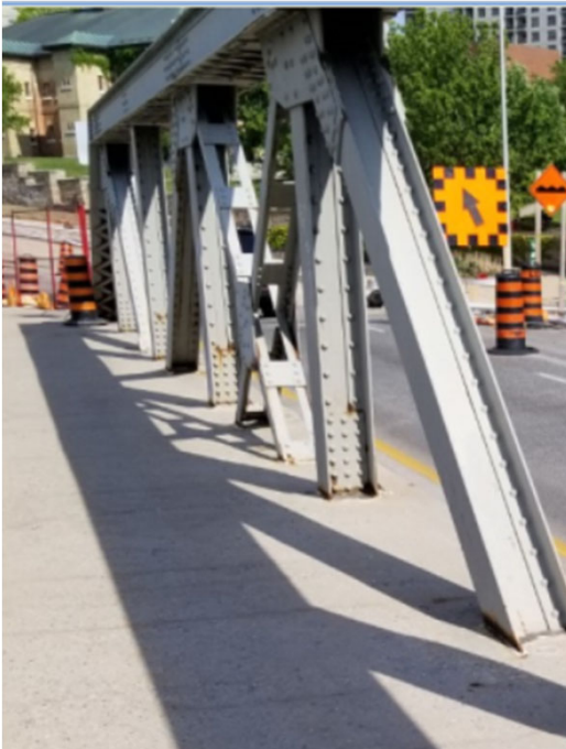
Kensington Bridge Truss
