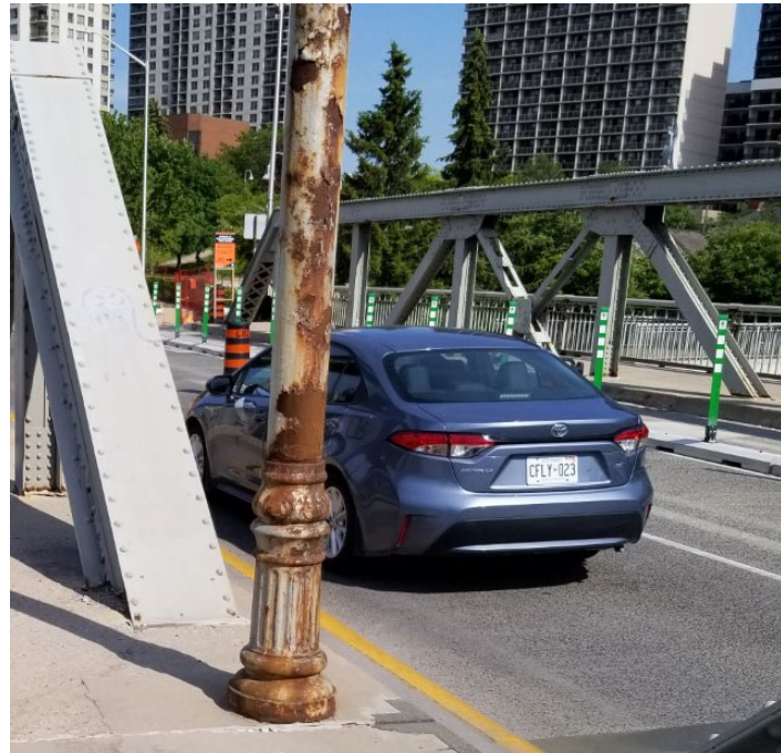
Kensington Bridge Existing Light Standard Base
