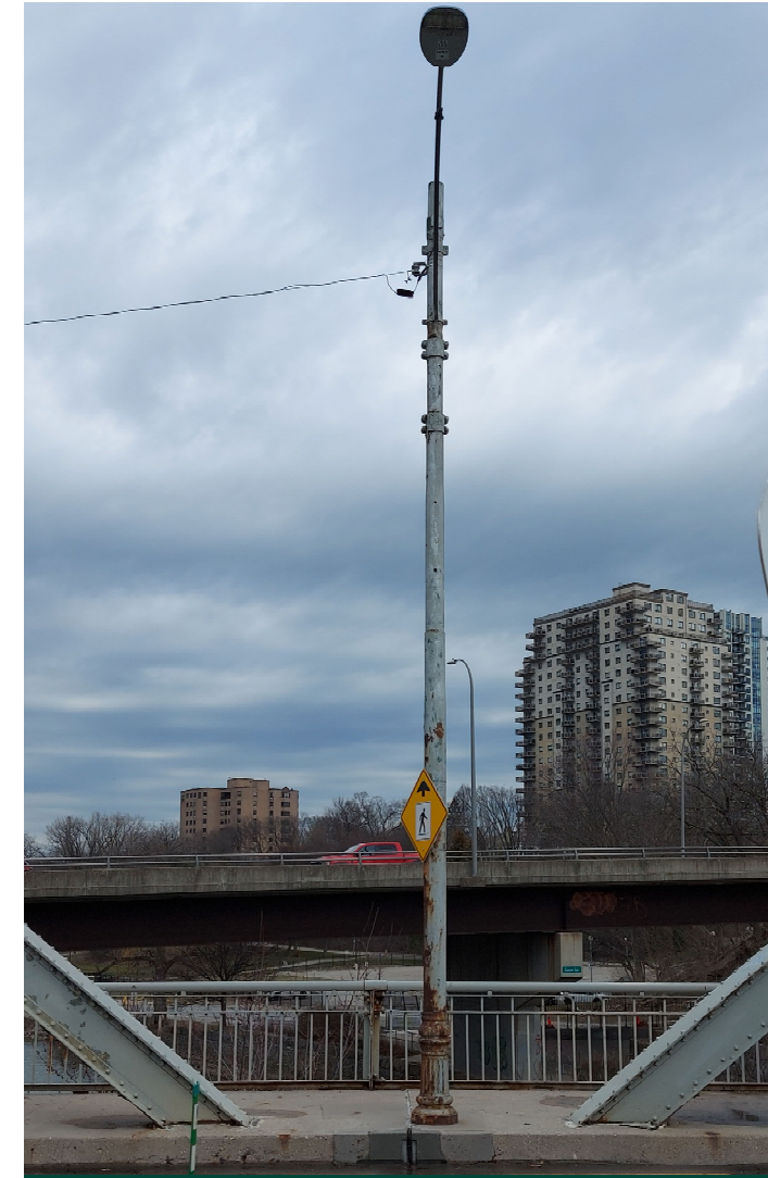
Kensington Bridge Existing Light Standard
