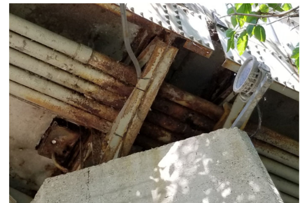
Kensington Bridge Soffit
