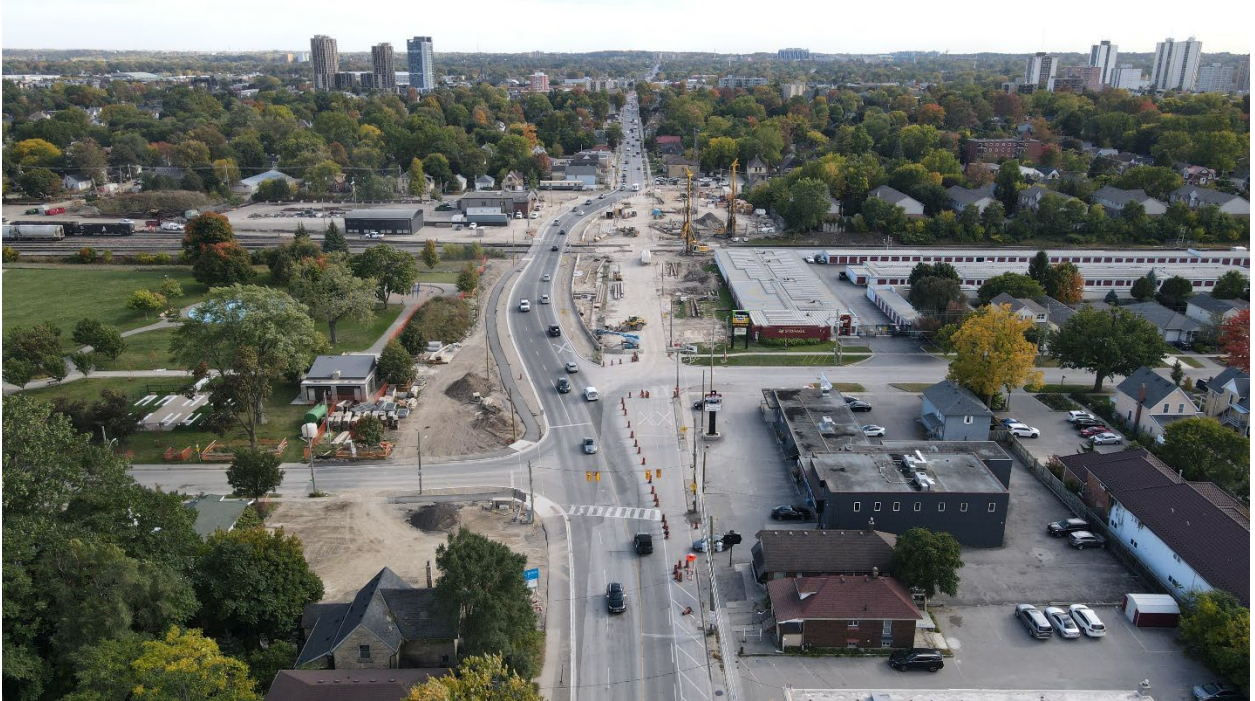
Above: Aerial view of the Adelaide Underpass construction site.
