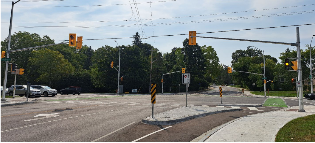
Above: New protected intersection at Ridout Street & Commissioners Road
