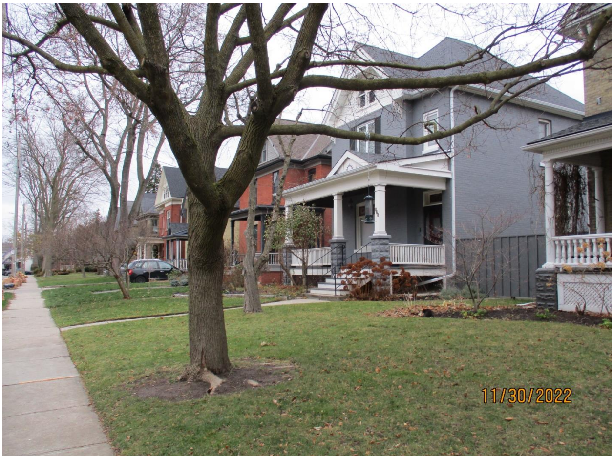
Image 2: Photograph showing the front yard of the property at 864 Hellmuth Avenue.
