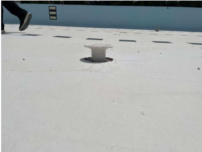
Photo 4 – Spalling of concrete along the crack line evident in the pool slab
