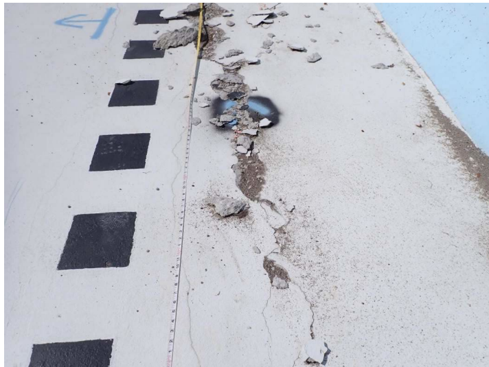
Photo 7 – Subgrade Deterioration
