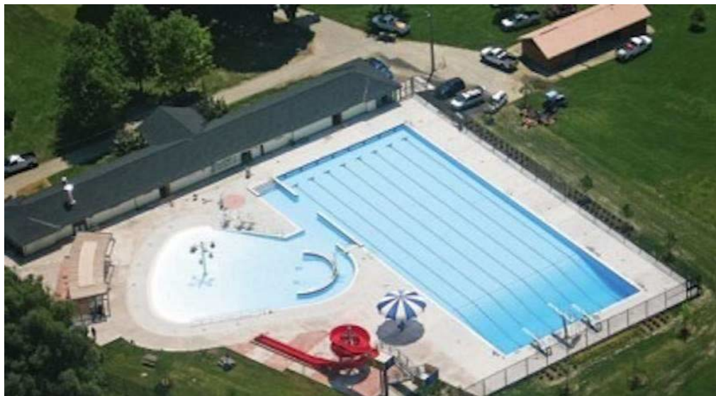
Photo 2 – Thames Pool Flooding 2018
