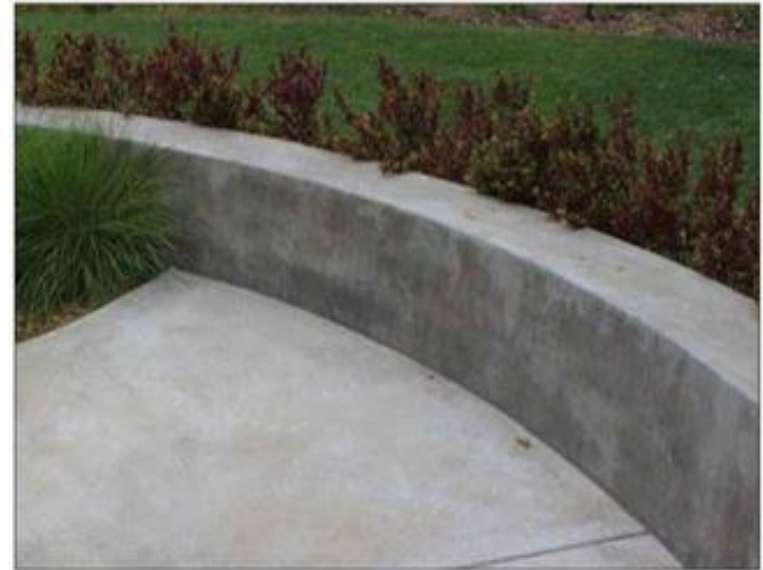
Example of concrete seat wall
