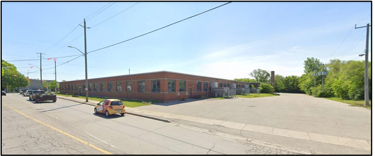
Figure 3. Streetview of 455 Highbury Avenue North (view from Brydges Street facing east)
