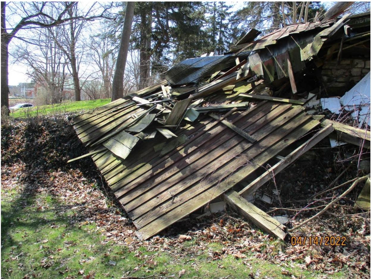
*Image 14: Photograph showing debris from the former accessory building, shown in April 2022. Note, a portion of the rubble stone foundation can be seen buried under the debris at right. A portion of the cherry board-and-batten exterior cladding can be seen at centre.*
