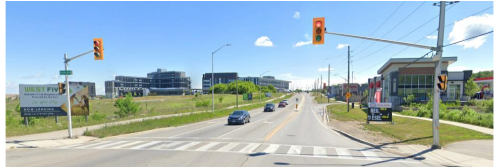
Oxford Street West at Westdel Bourne, looking east
