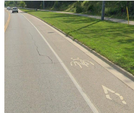
Existing On-Road Cycling Lanes
