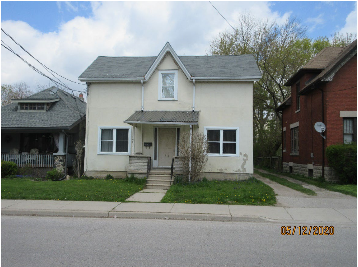
Image 1: Photograph of the subject property at 19 Blackfriars Street, within the Blackfriars/Petersville Heritage Conservation District prior to the installation of the new vinyl siding (2020).
