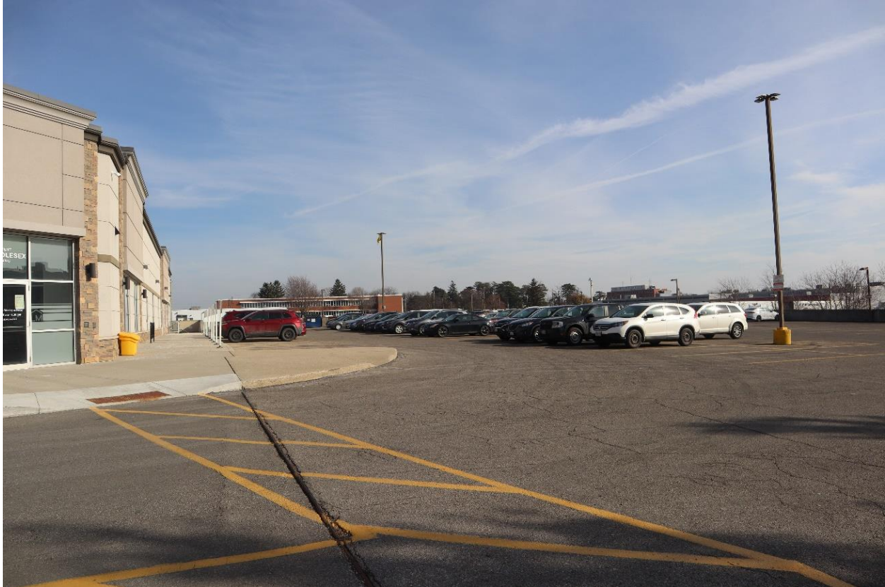
Photo 4: View of the Development Area showing the concrete sidewalk and parking lot, with the Study Area (955 Highbury Avenue North) visible in the background (AECOM, November 2022)
