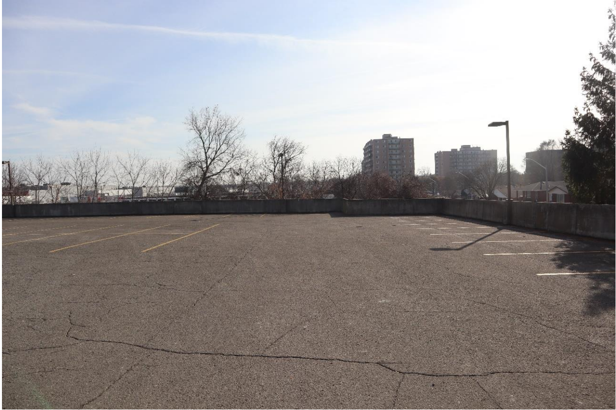
Photo 5: View of the Development Area showing the parking lot atop the parking garage (AECOM, November 2022)
