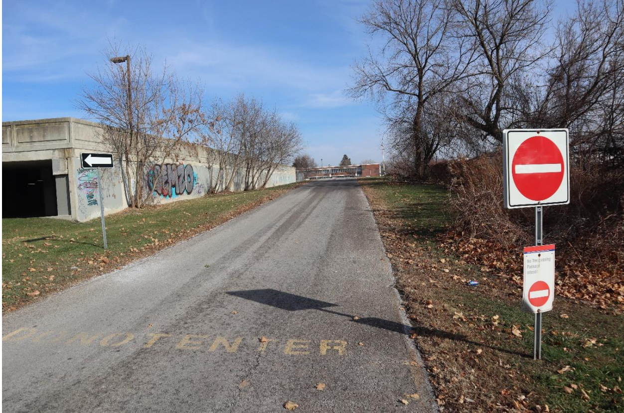
Photo 2: View of the enclosed parking garage and private asphalt road, with the Study Area (955 Highbury Avenue North) visible in the distance (AECOM, November 2022)
