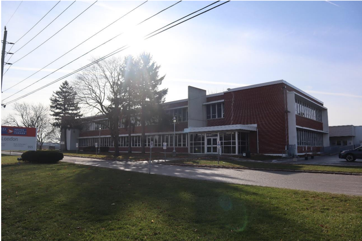
Photo 8: View of the east elevation of the Study Area (955 Highbury Avenue North) from the right-of-way (AECOM, November 2022)
