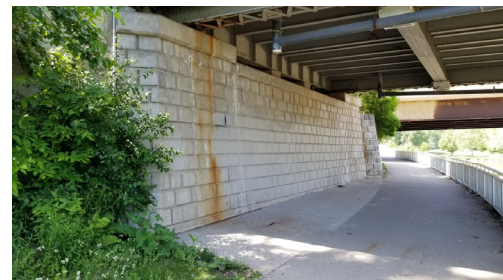
TVP passing under the west side of the Kensington Bridge
