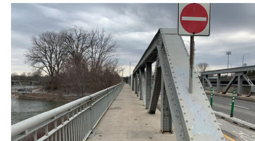
Existing pedestrian walkway on Kensington Bridge
