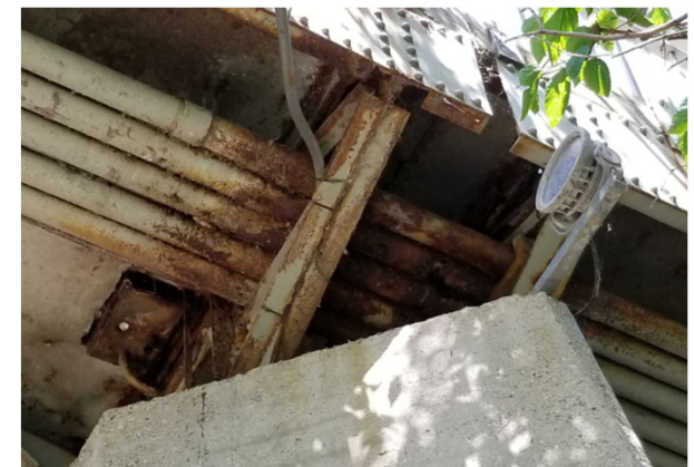
Kensington Bridge Soffit
