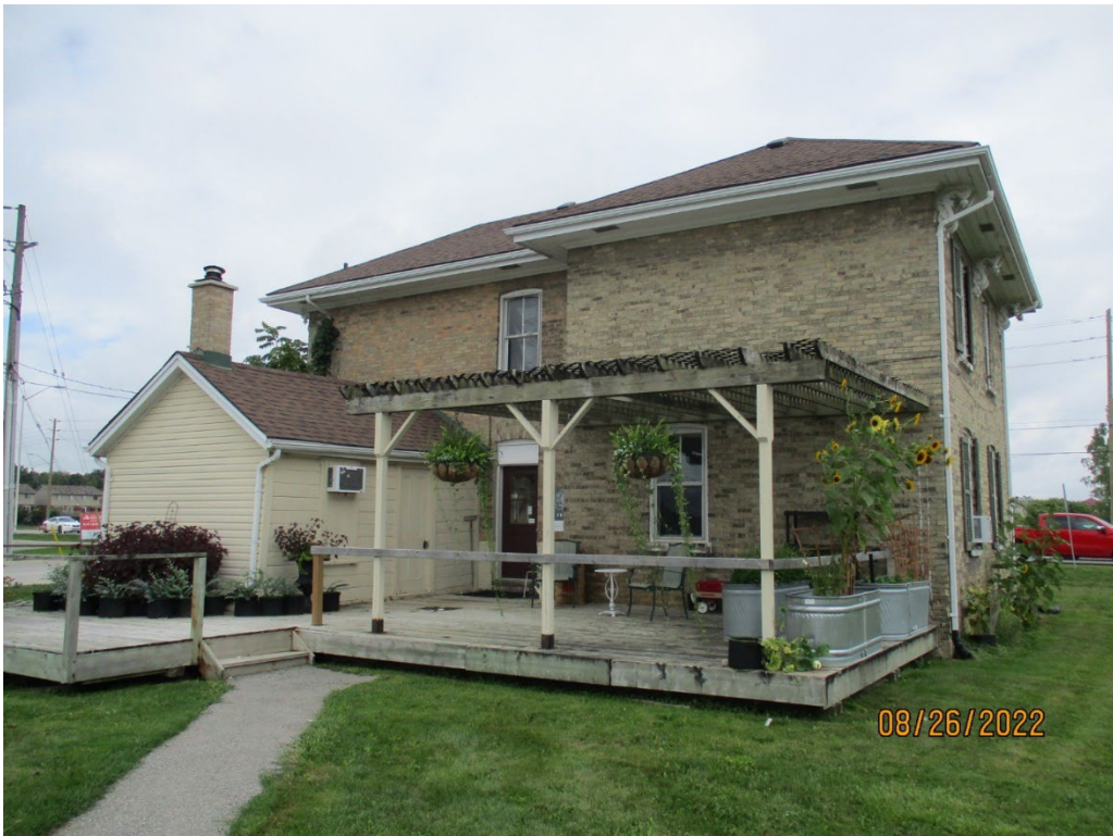
Image 14: Photograph showing the rear (west) façade of the Routledge Farmhouse at 1656 Hyde Park Road, August 26, 2022.
