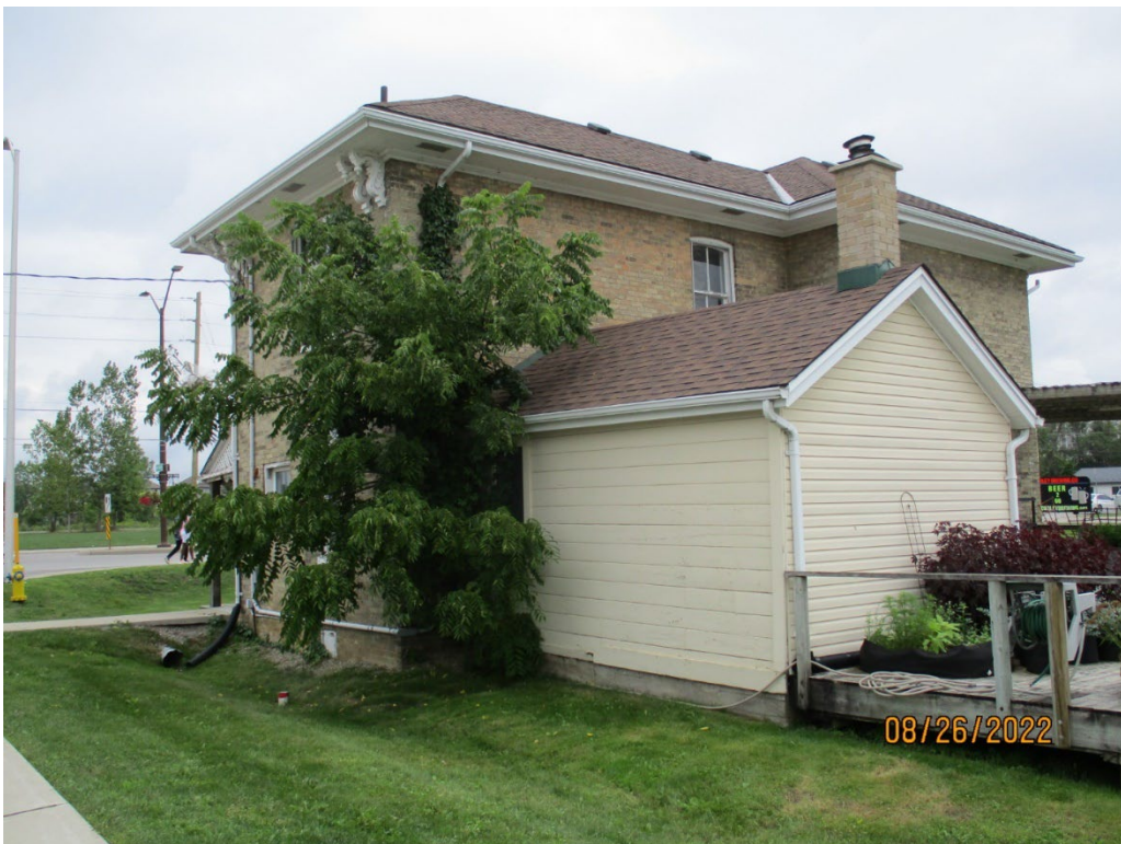
Image 16: Photograph showing the rear (west) façade of the Routledge Farmhouse at 1656 Hyde Park Road, August 26, 2022.
