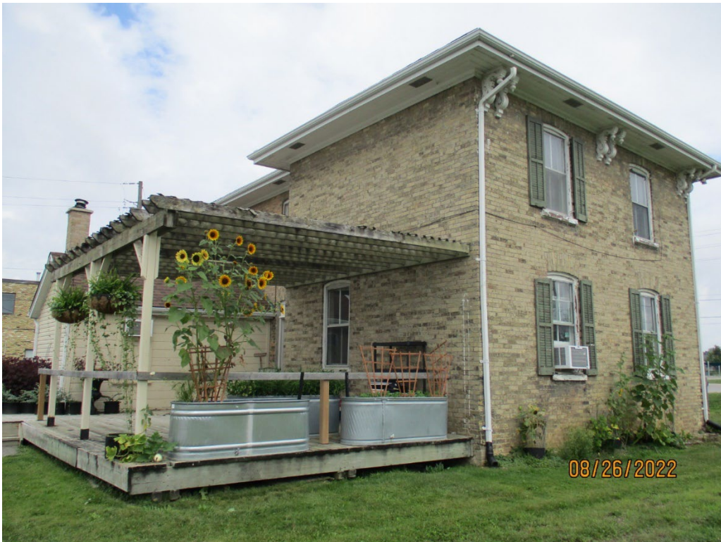
Image 12: Photograph looking north east showing the rear (west) façade at left and south façade at right, August 26, 2022.
