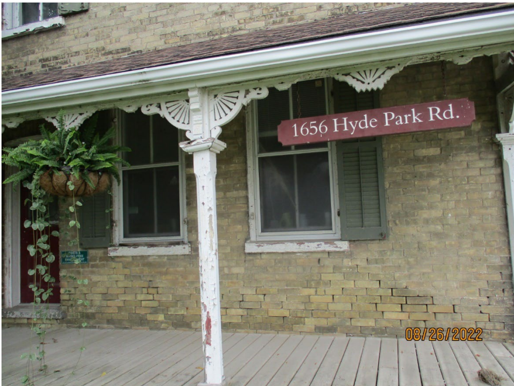
Image 4: View showing the chamfered posts with capitals and fretwork on the existing porch on the Routledge Farmhouse at 1656 Hyde Park Road, August 26, 2022.
