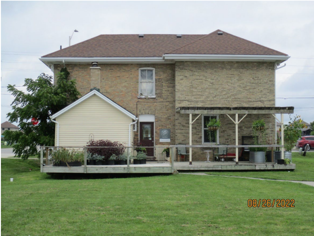
Image 15: Photograph showing the rear (west) façade of the Routledge Farmhouse at 1656 Hyde Park Road, August 26, 2022.
