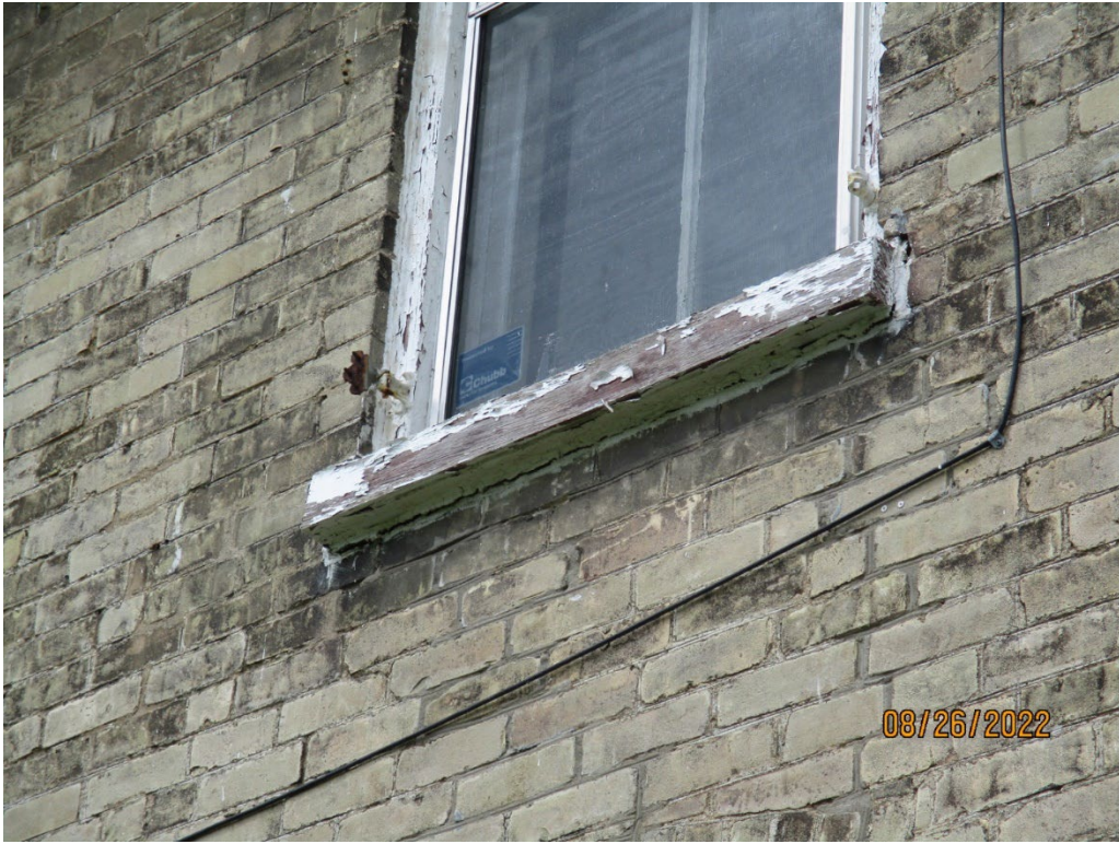
Image 11: Detail showing buff brick and existing wood sills on the Routledge Farmhouse at 1656 Hyde Park Road, August 26, 2022.
