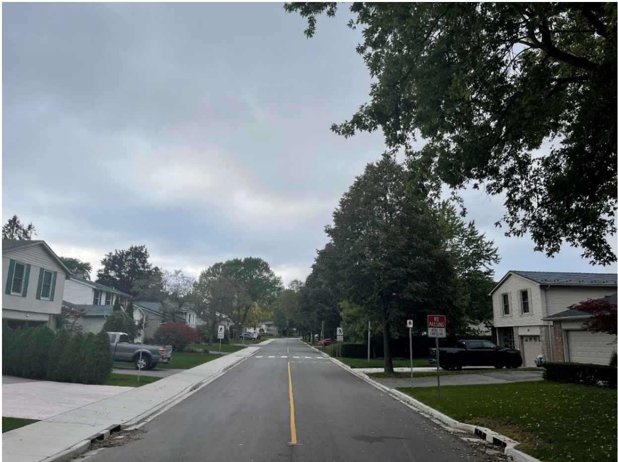
Figure 1: Photo of a completed Local Road Reconstruction Program with a new sidewalk
