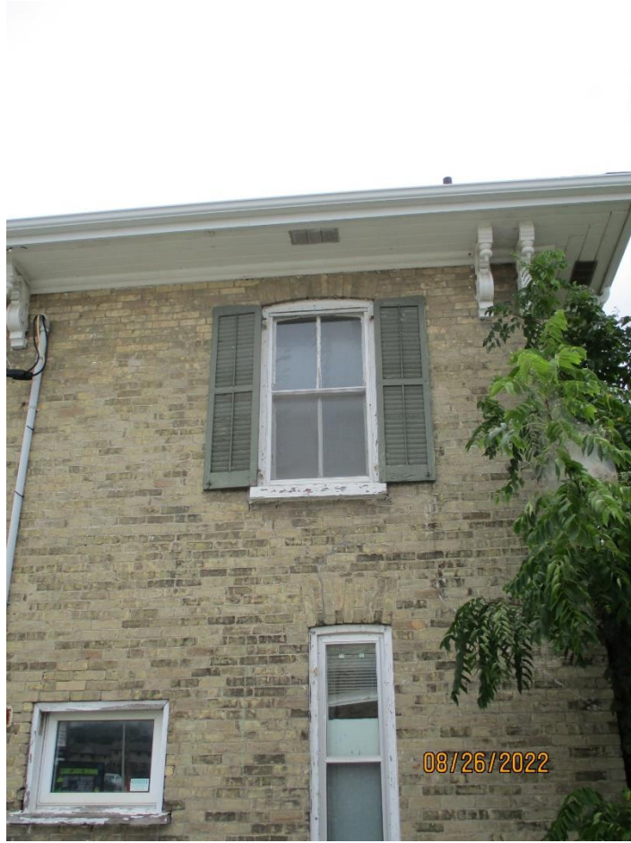
Image 18: Photograph looking south showing the north façade of the Routledge Farmhouse, August 26, 2022.
