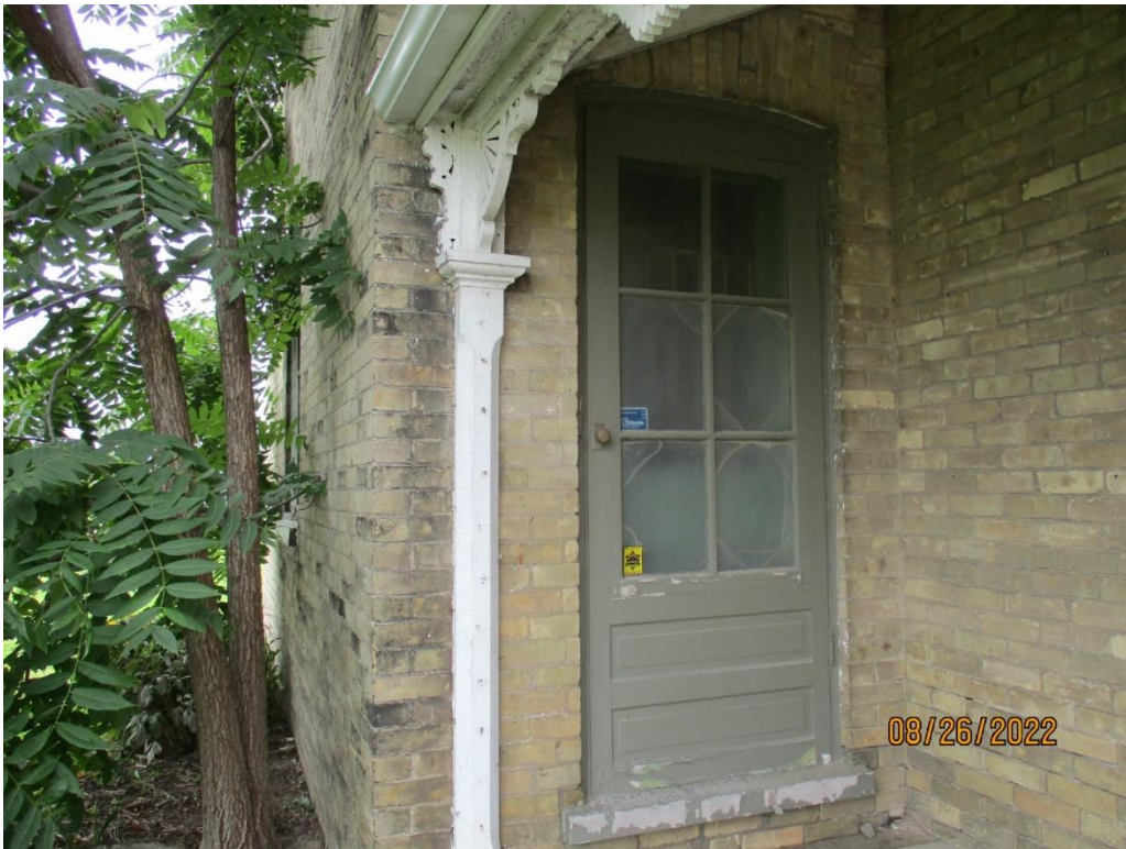
Image 6: Photograph showing the wooden door located at the south end of the porch entry door on of the Routledge Farmhouse, August 26, 2022.
