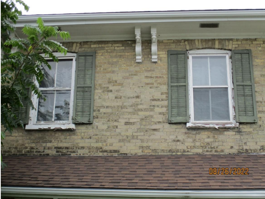
Image 3: View showing the existing double-hung wood windows, with wood shutters, as well as the deep eaves and paired brackets on the Routledge Farmhouse, August 26, 2022.
