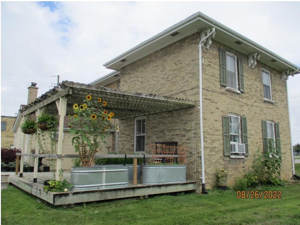
Image 12: Photograph looking north east showing the rear (west) façade at left and south façade at right, August 26, 2022.
