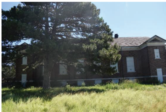
Photo 19: Recreation Hall west elevation looking east
