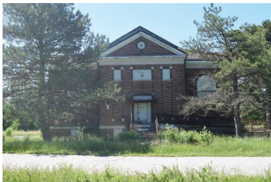
Photo 18: Recreation Hall front (north) elevation looking south
