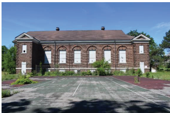
Photo 20: Recreation Hall east elevation looking west
