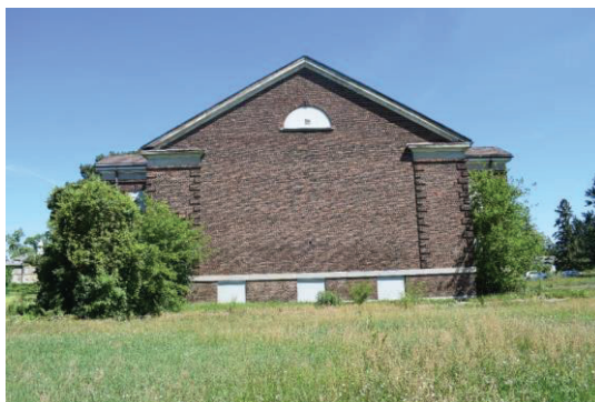
Photo 21: Recreation Hall south elevation looking north
