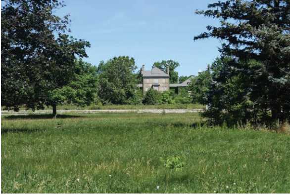
Photo 30: Open space to the south of the Infirmary looking northeast
