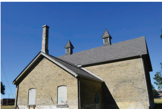
Photo 5: Horse Stable looking southwest
