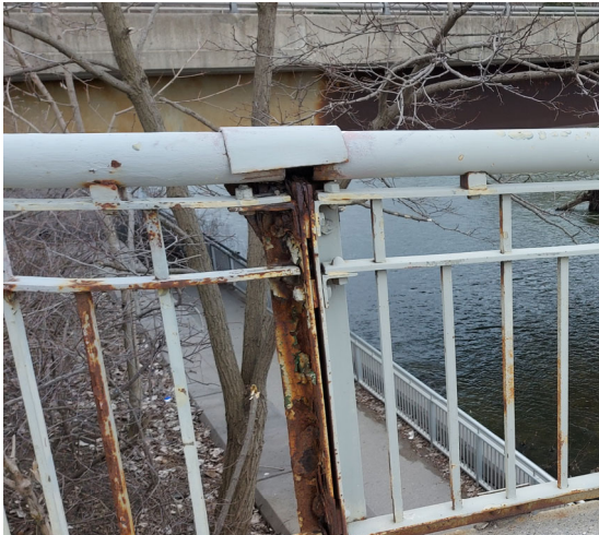
15 Kensington Bridge Existing Railing
