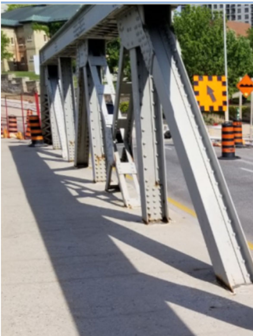
Kensington Bridge Truss
