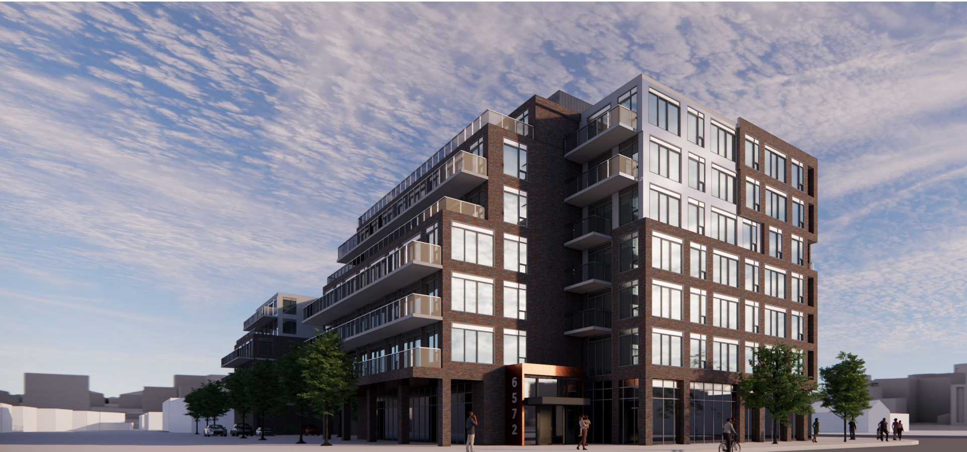
South Façade from Dundalk Dr.
