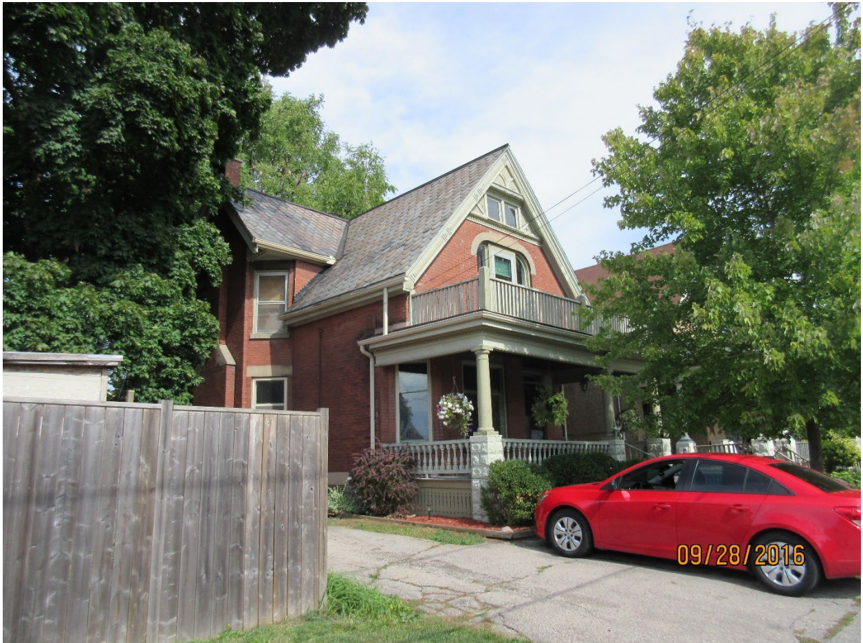
Image 1: Photograph showing the dwelling located at 892 Princess Avenue, showing original slate roof (2016).
