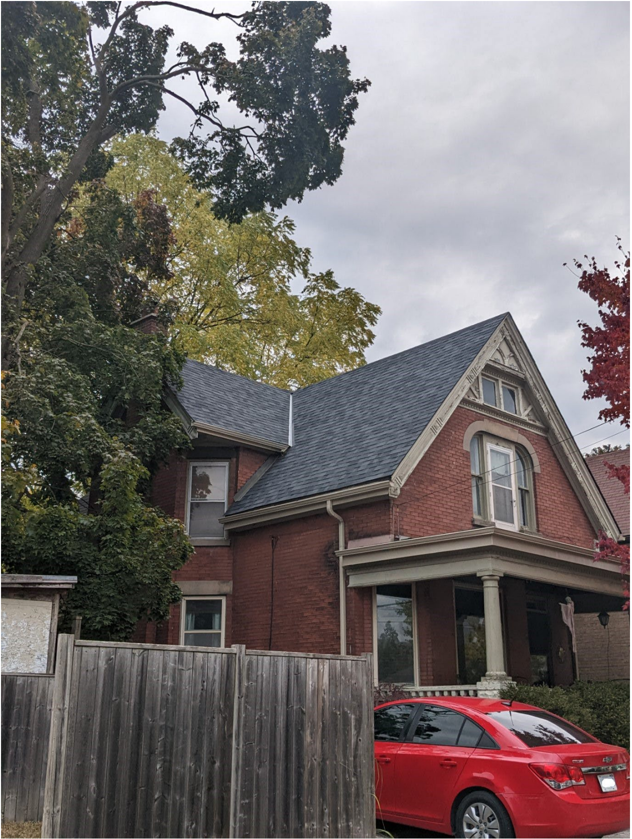
Image 5: Photograph submitted as a part of the pre-consultation process for the Heritage Alteration Permit application showing the unapproved asphalt shingles.
