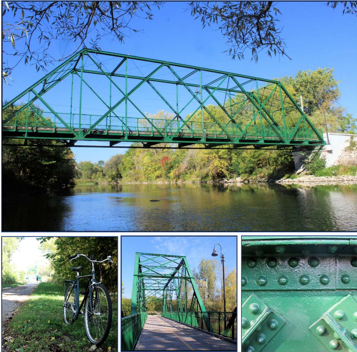
26. (top) Meadowlily Bridge main span viewed from the south east bank of the Thames River.
