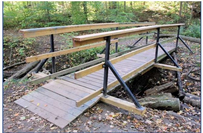
43. Walking trail bridge in Meadowlily Woods ESA.
