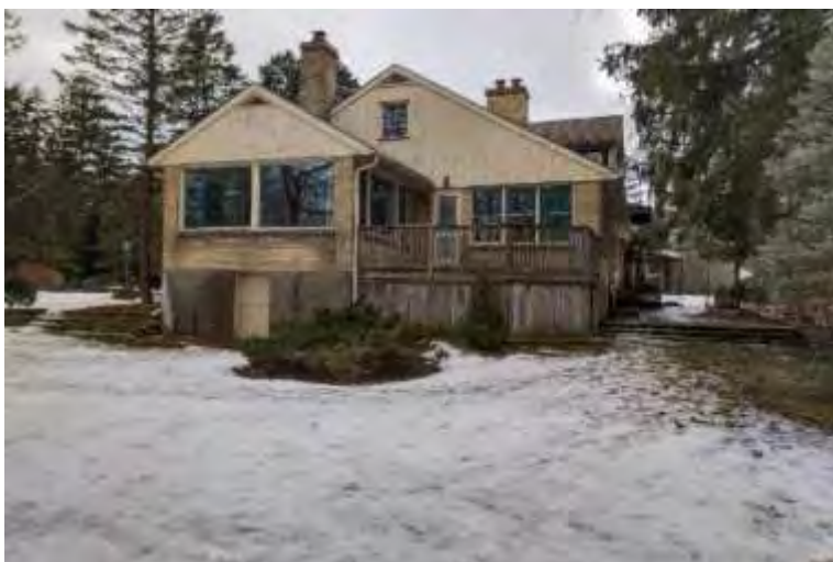
Photo 10: Existing house (back view) and backyard
