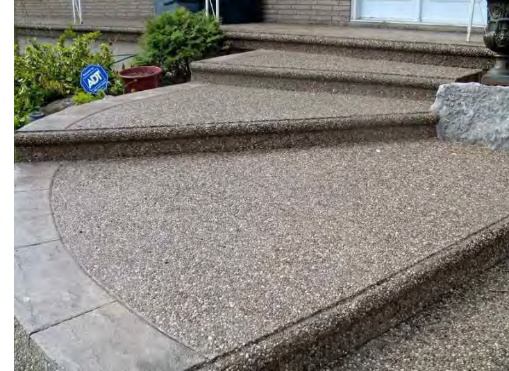
1. EXPOSED AGGREGATE CONCRETE STEPS AND DRIVEWAY WITH 8" CONCRETE BANDING AROUND PERIMETER
