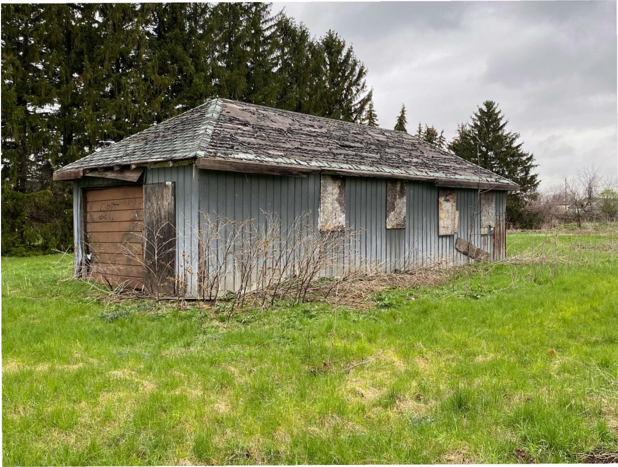
Image 1. Garage (B12001), facing northeast – L. Dent, May 2022
