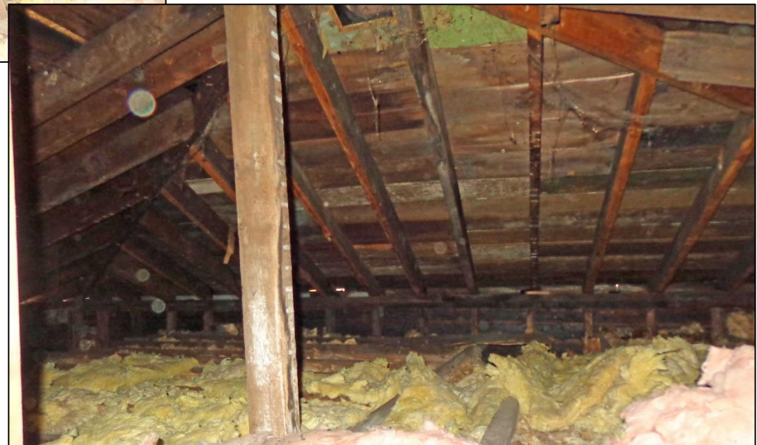
4. Attic – Tail Wing – View West.
