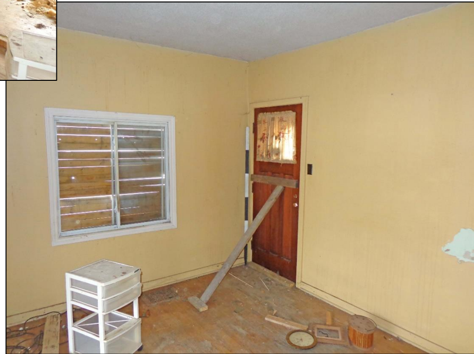
8. Room 3 – South and West Walla and Door to Outside.
