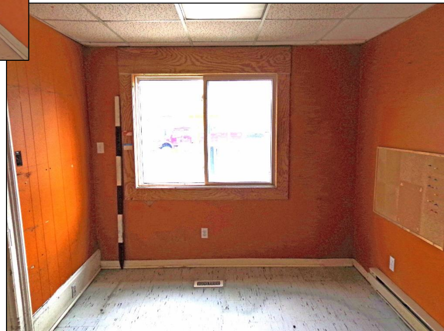
8. Room 2 – North, East and South Walls.
