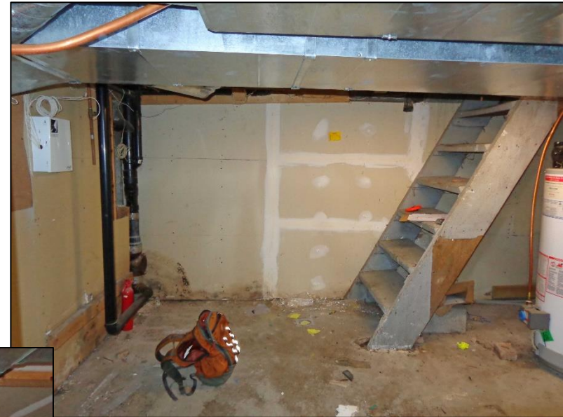
1. Room 1 – East and South Walls.
