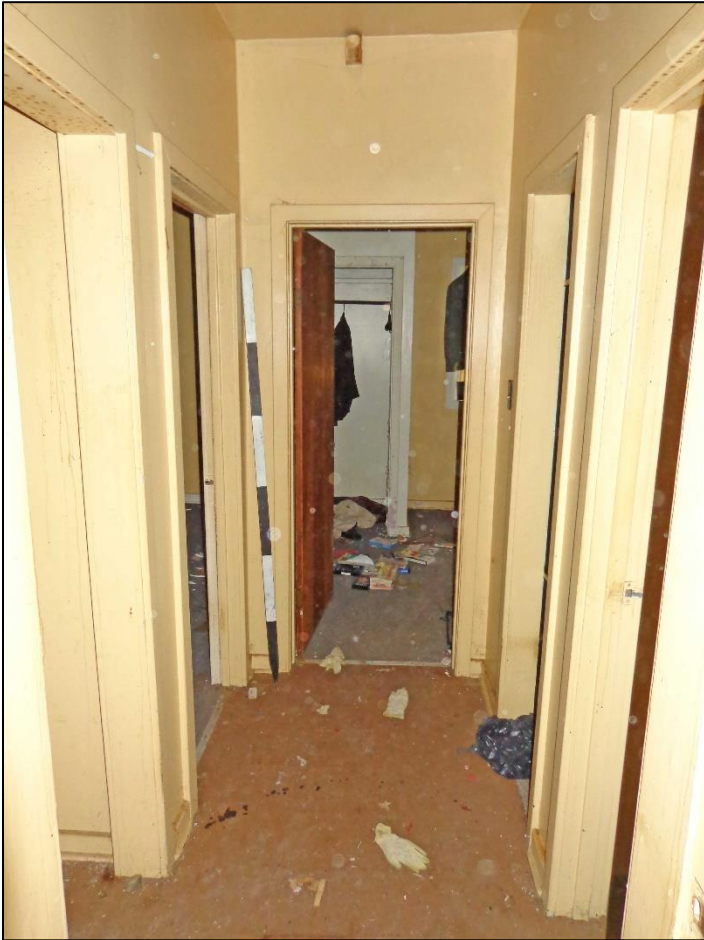
15. Hall – View West to Room 6.
