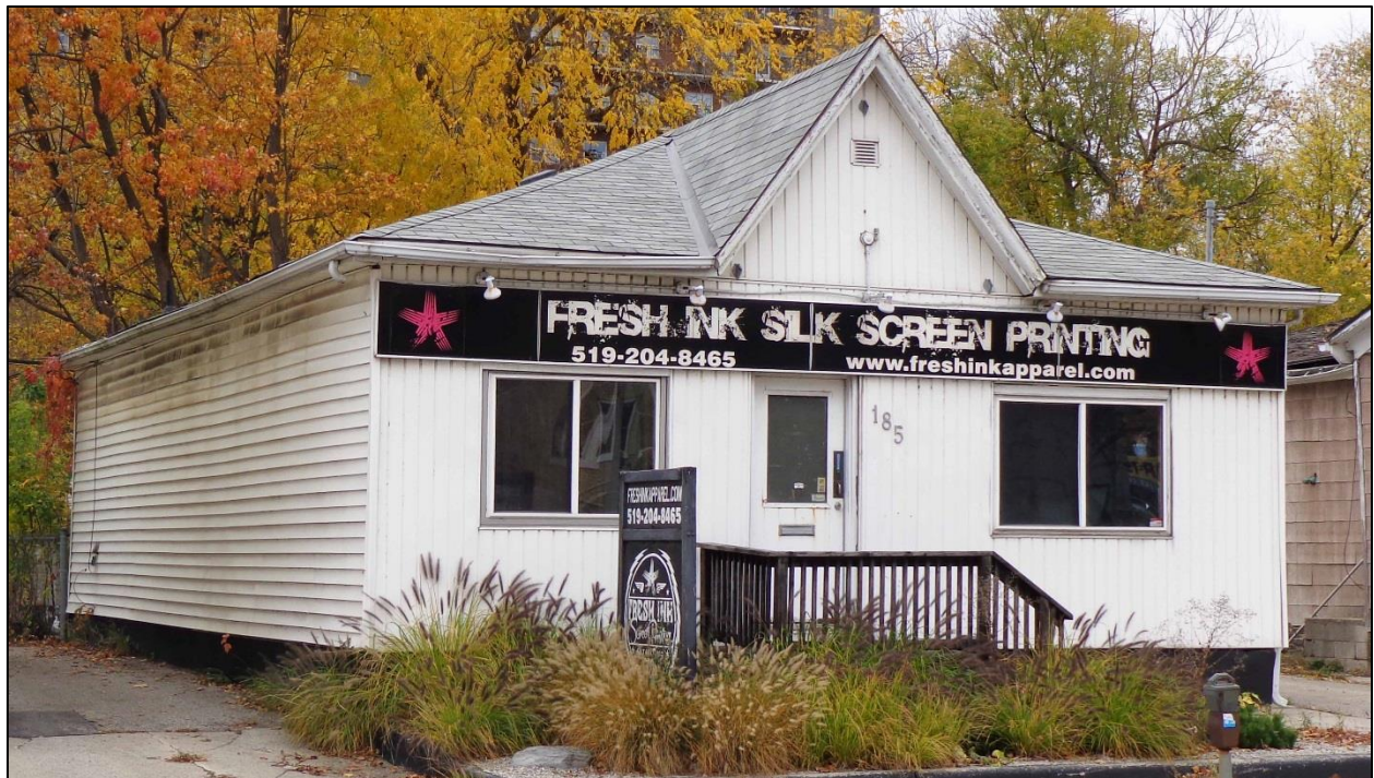
South and East Elevations
