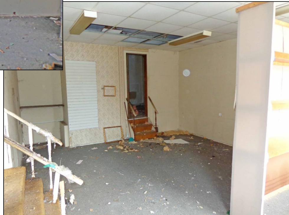
4. Room 1 – West and North Wall and Entrance to Room 8.
