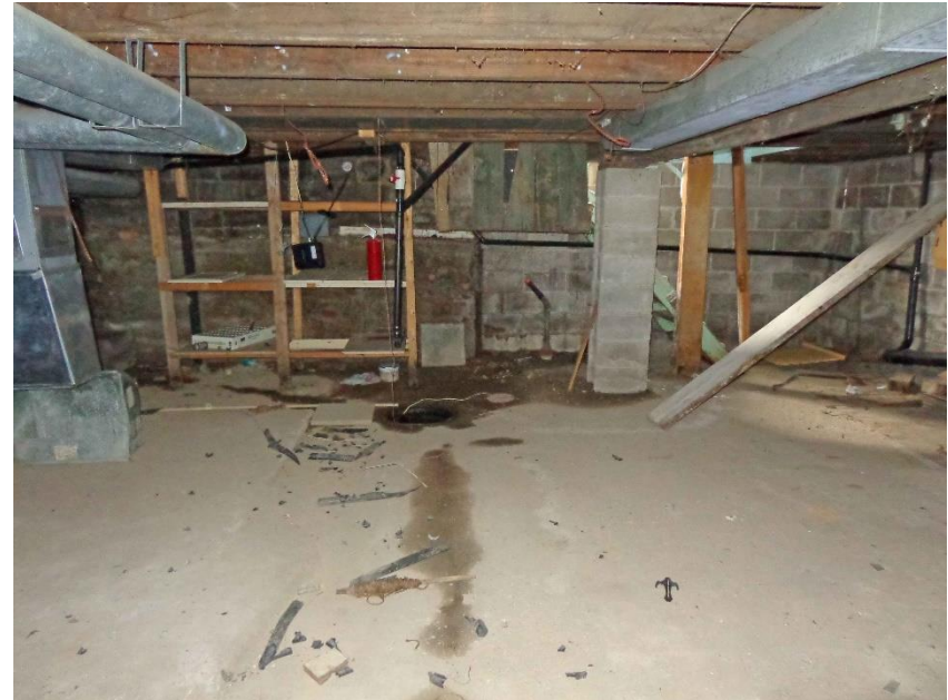
1. Room 1 – South Wall and Staircase up.
