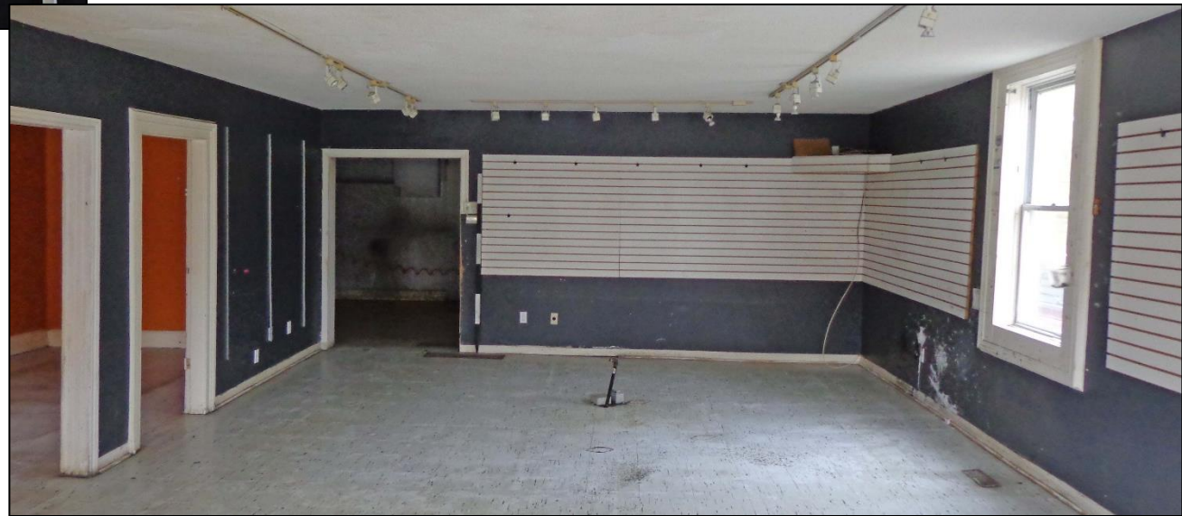
6. Room 1 – South, West and North Walls.
