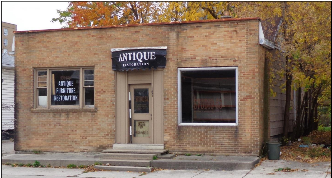
East and North Elevations
