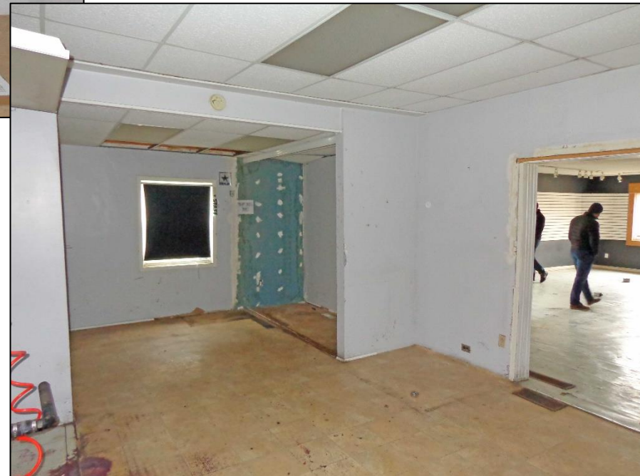
15. Room 4 – North and East Walls.
