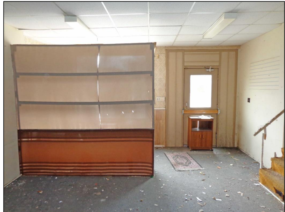
1. Room 1 – North, East and South Walls.
