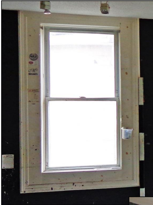
5. Room 1 – Window, North Wall, Detail - new mouldings.
