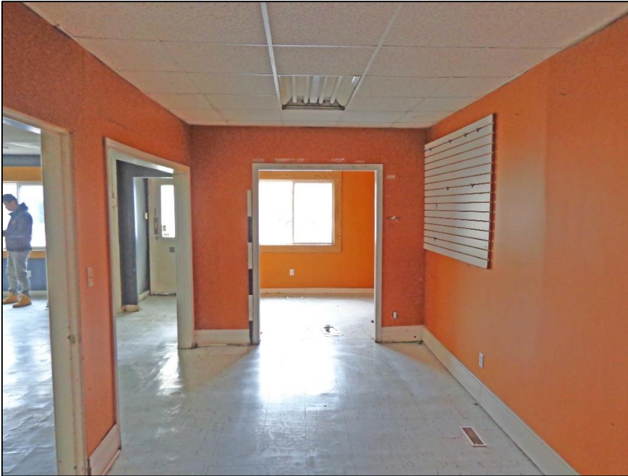
12. Room 3 – North, East and South Walls.
