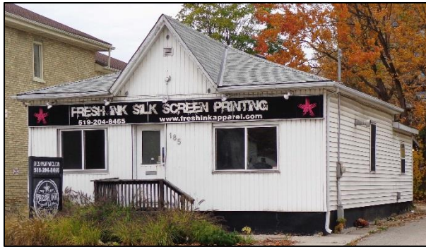
185 - East and North Elevations
