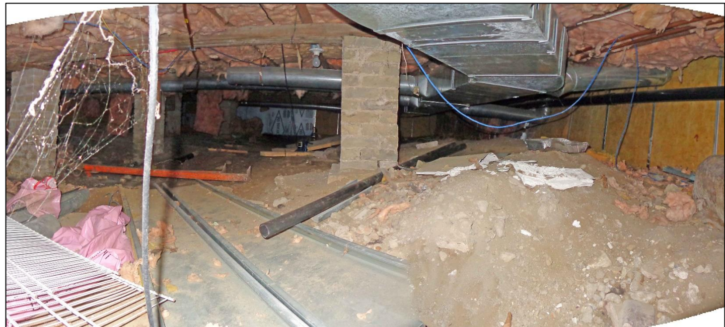
6. Crawl Space – View East and South from Room 1 access.
