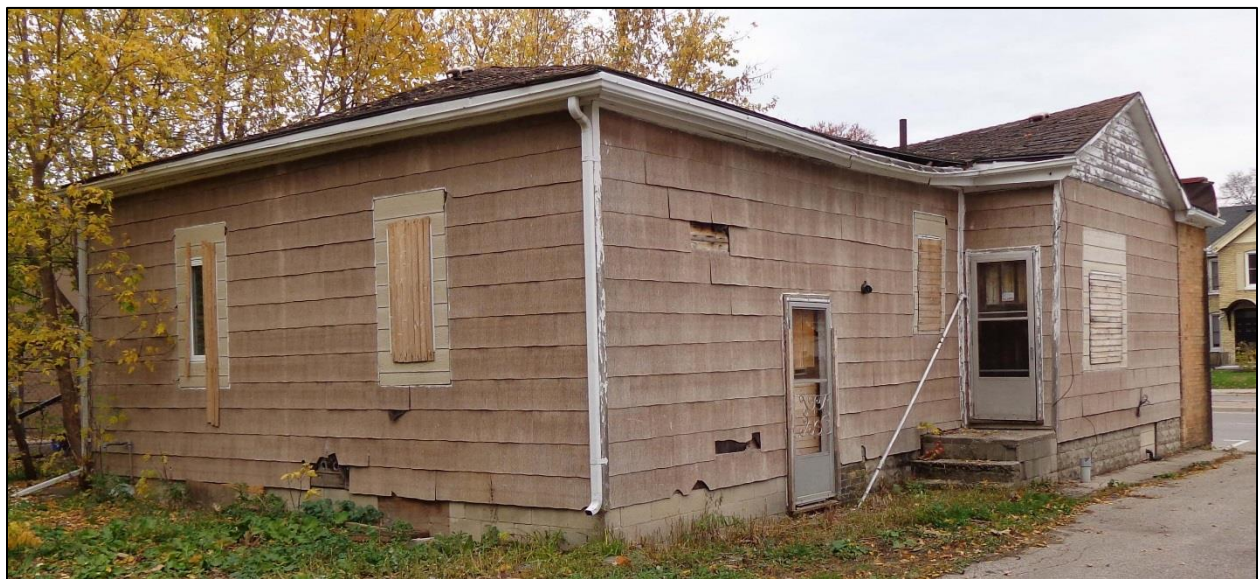
West and South Elevations
