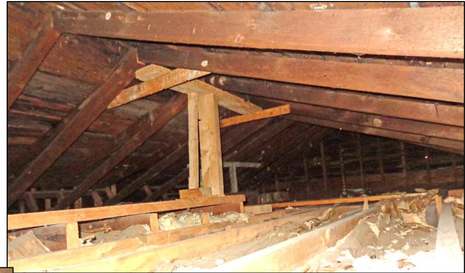
2. Attic – Front Section – View East and South.
