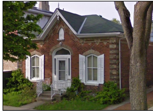
Figure 5.2 108 Albion Street, Brantford. [Source: Google Street view, 2012].
