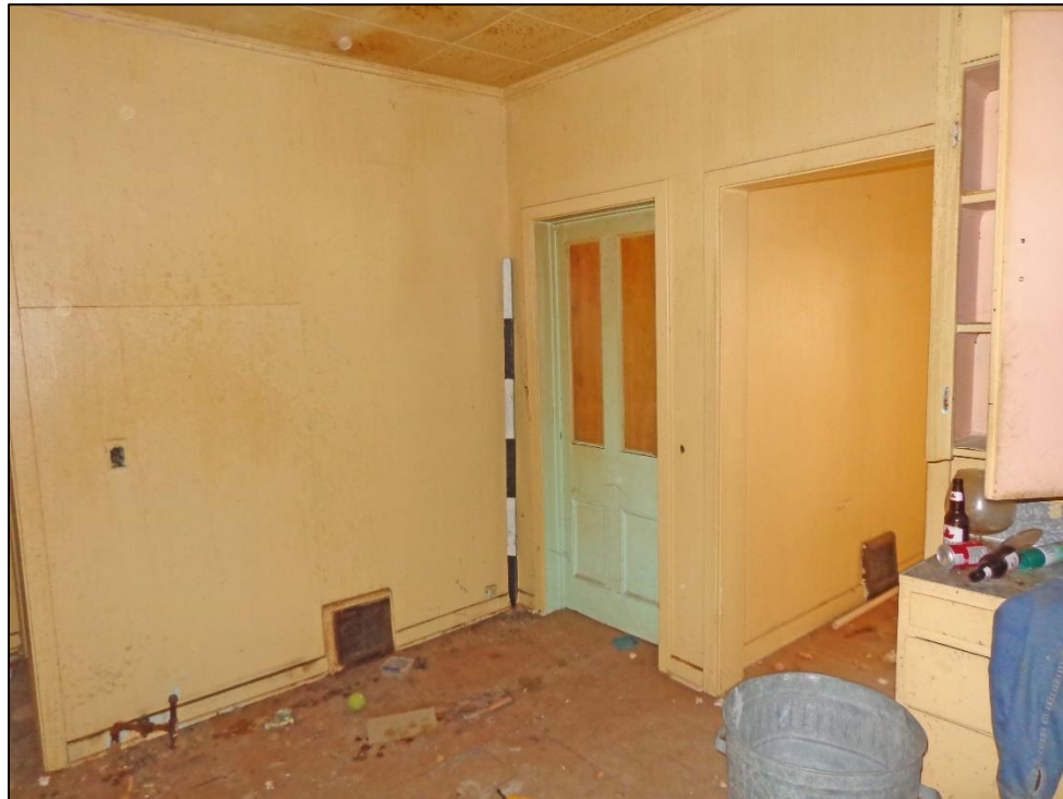
9. Room 4 – North and East Wall and opening to Room 3.
