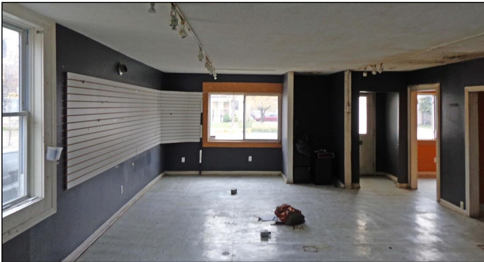
2. Room 1 – North, East and South Walls.
