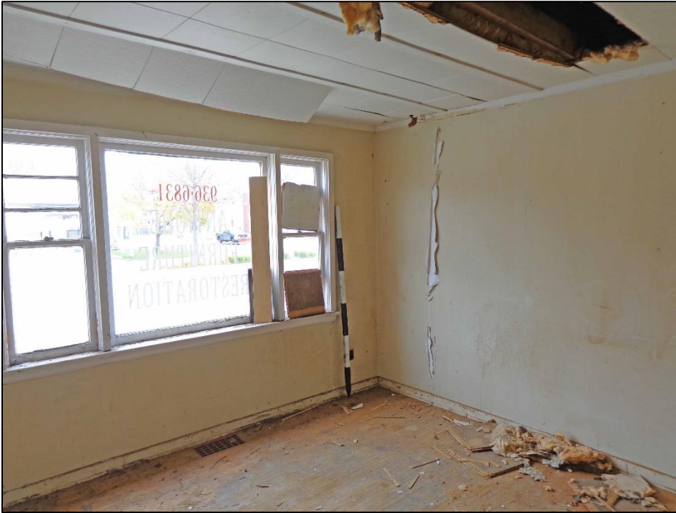
5. Room 2 – East and South Walla.
