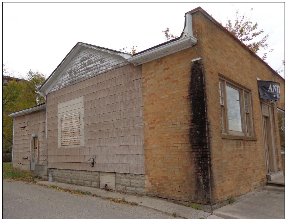
South and East Elevations
