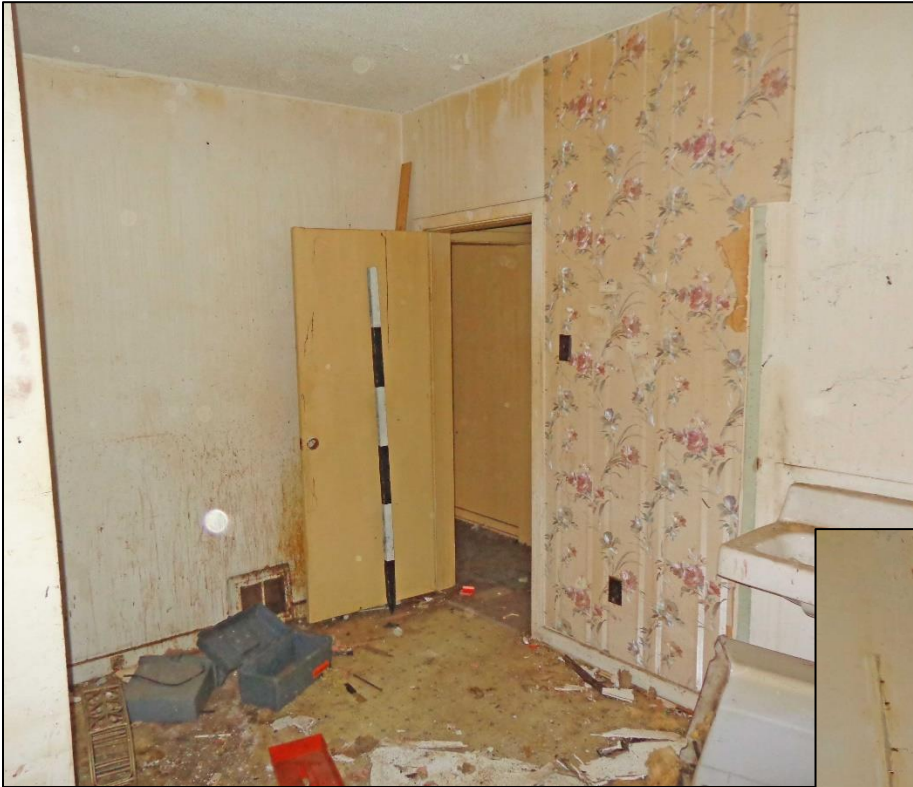
19. Room 8 – South and West Walls and Door to Hall.
