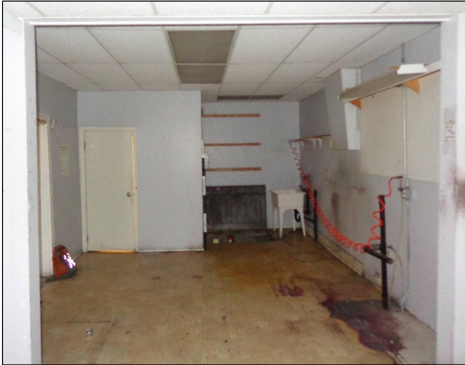
16. Room 4 – East, South and West Walls.
