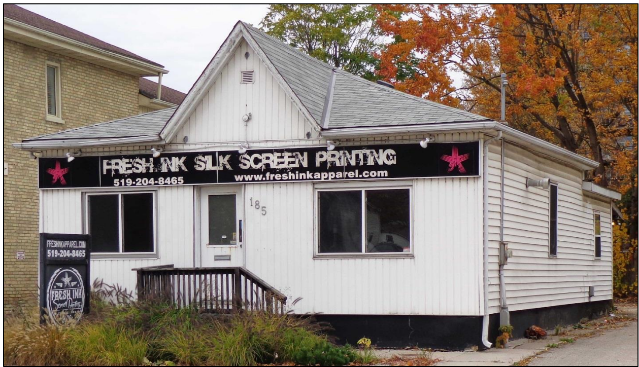
East and North Elevations
