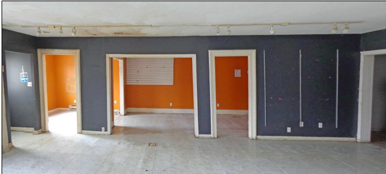
3. Room 1 – South Wall.
