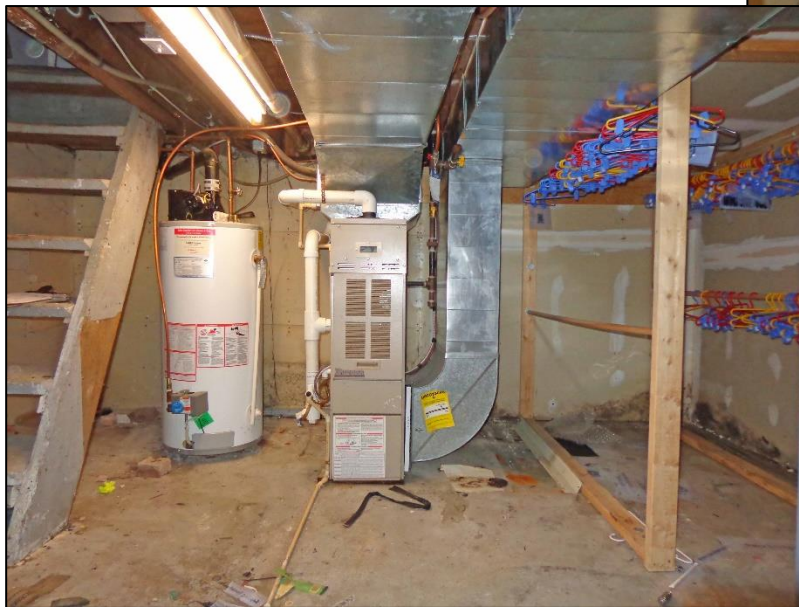
2. Room 1 – West and North Walls.
