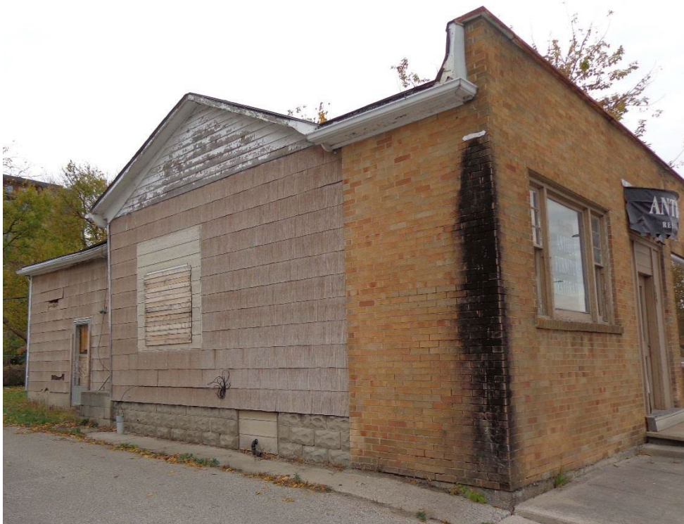
Image 5. 189 Wellington Street, façade detail-facing northeast – W. Morgan (CHIS, Jan 2021)
