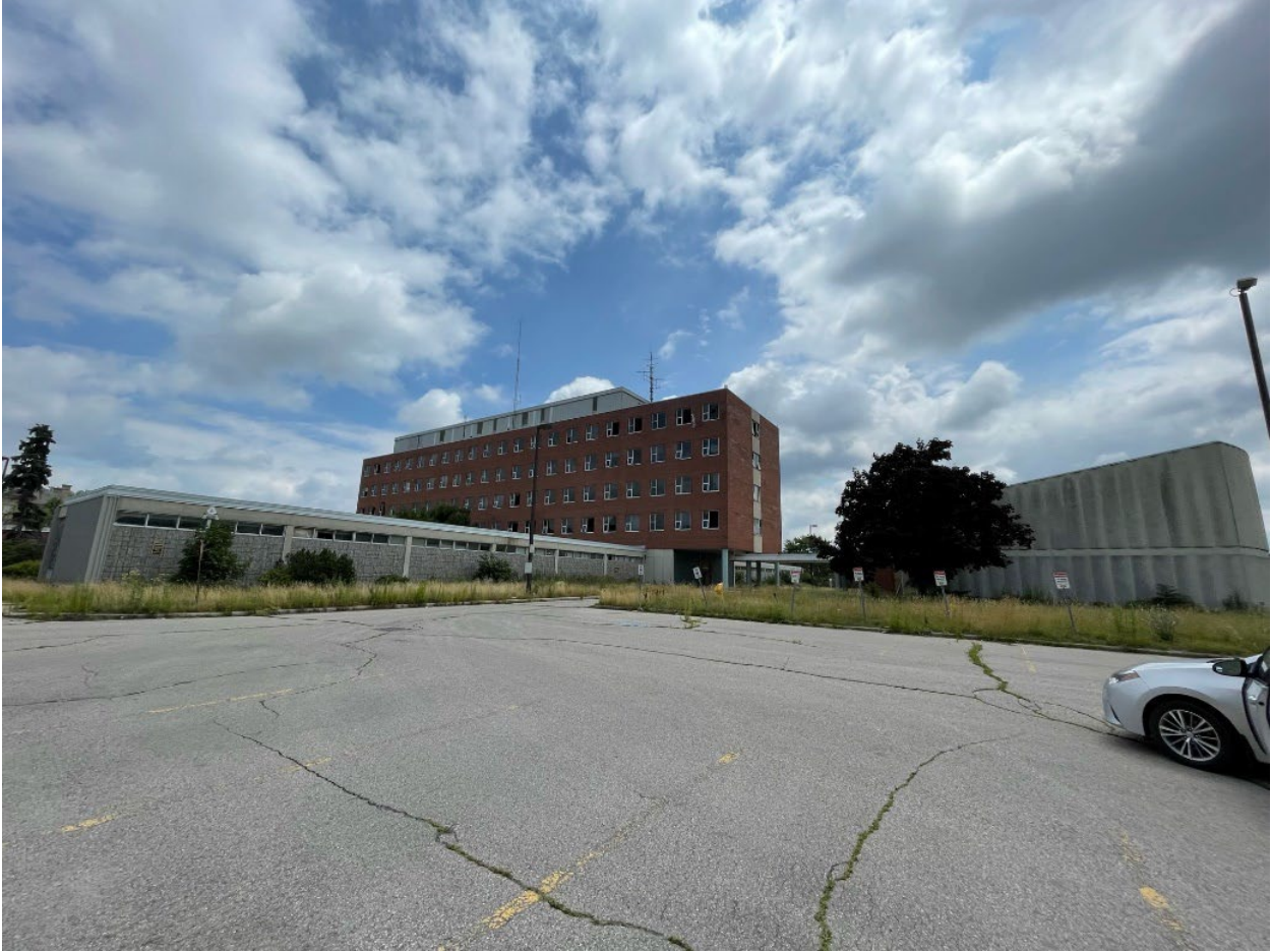
Image 6. South Pavilion Building and Extensions – as noted on project plan (including B12007, B12008, and B12012), facing southeast – Old Oak Properties, July 2022
