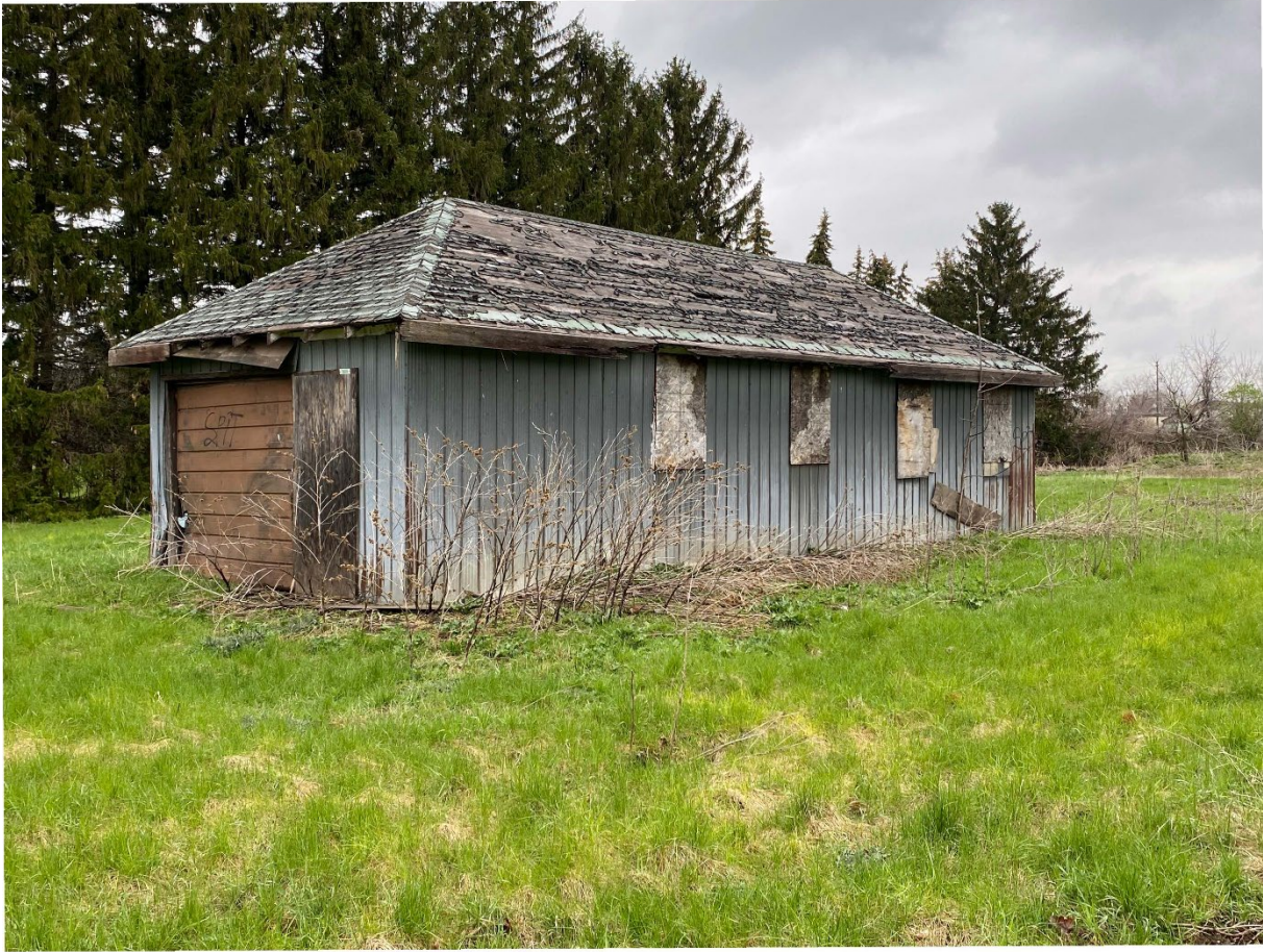
Image 1. Garage (B12001), facing northeast – L. Dent, May 2022
