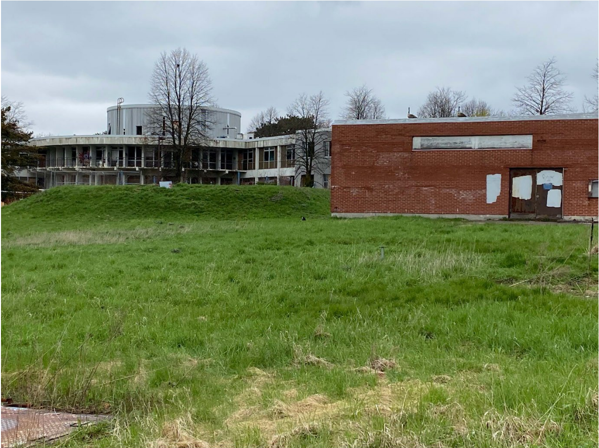
Image 3. Pump House & Underground Water Storage Tank (B12015, B16184), facing northwest – L. Dent, May 2022
