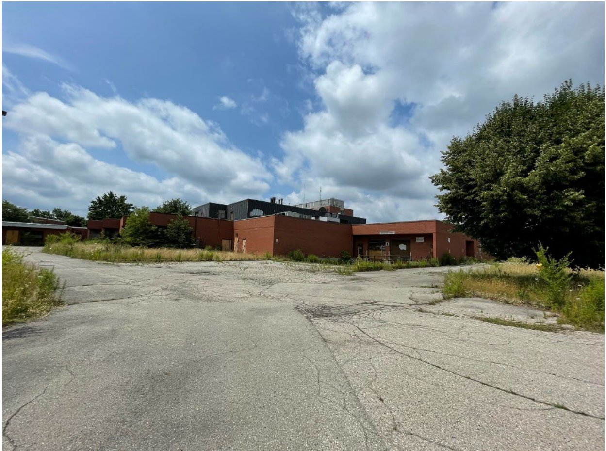
Image 8. South Pavilion Building and Extensions – as noted on project plan (including B20794, B12009, and B12014), facing southwest – Old Oak Properties, July 2022
