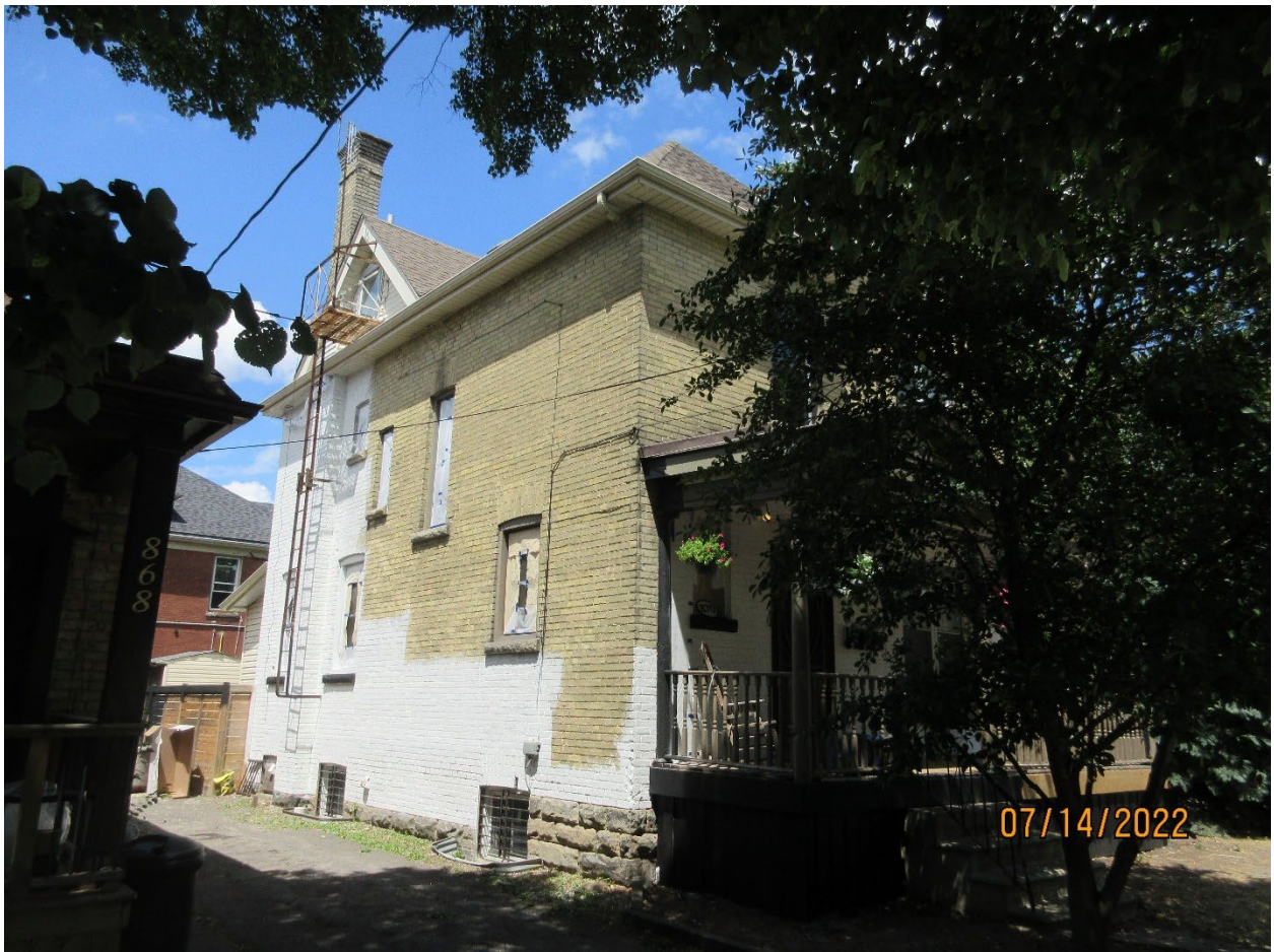
Image 6: Photograph of the heritage designated property at 870 Queens Avenue, on July 14, 2022, showing painting on the west façade.
