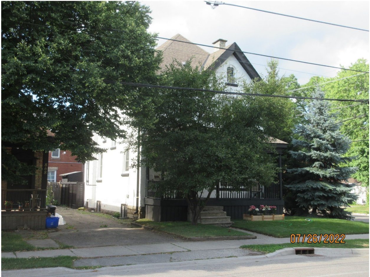
Image 8: Photograph of the heritage designated property on July 26, 2022, showing that the west façade of the building has been painted.
