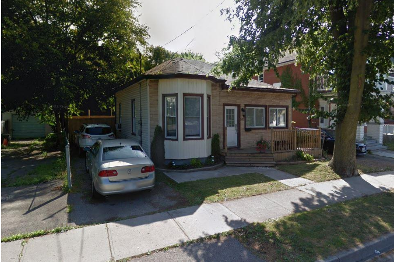
Image 1: Google Street Image of the dwelling on the subject property at 520 Ontario Street, shown in August 2019, prior to experiencing damage.
