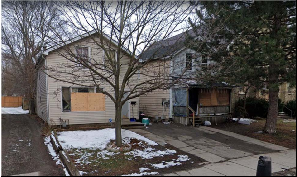
Figure 19: 142 Wellington Street (left), 140 Wellington Street (right)
