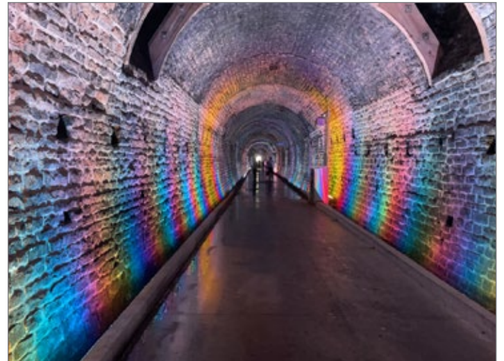
Brockville Rail Tunnel
