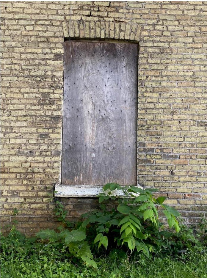
Image 14: Detail of boarded-up window opening – 1<sup>st</sup> floor, west elevation – showing shallow arch with voussoirs and two-over-two (2/2) wooden window frame and wood sill
