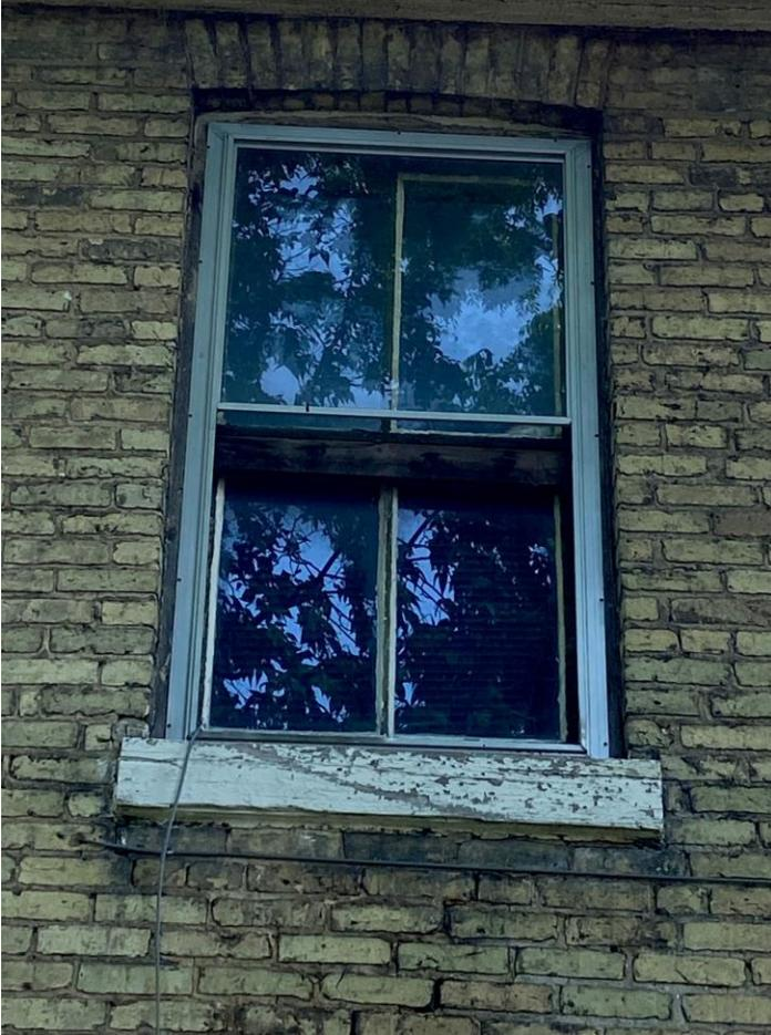
Image 13. Detail of window opening – 2<sup>nd</sup> floor, west elevation – showing shallow arch with voussoirs and two-over-two (2/2) wooden window frame and wood sill
