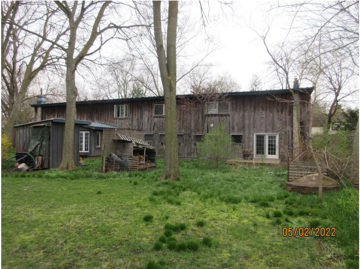
Image 3: View of the east façade of the building at 514 Pall Mall Street.
