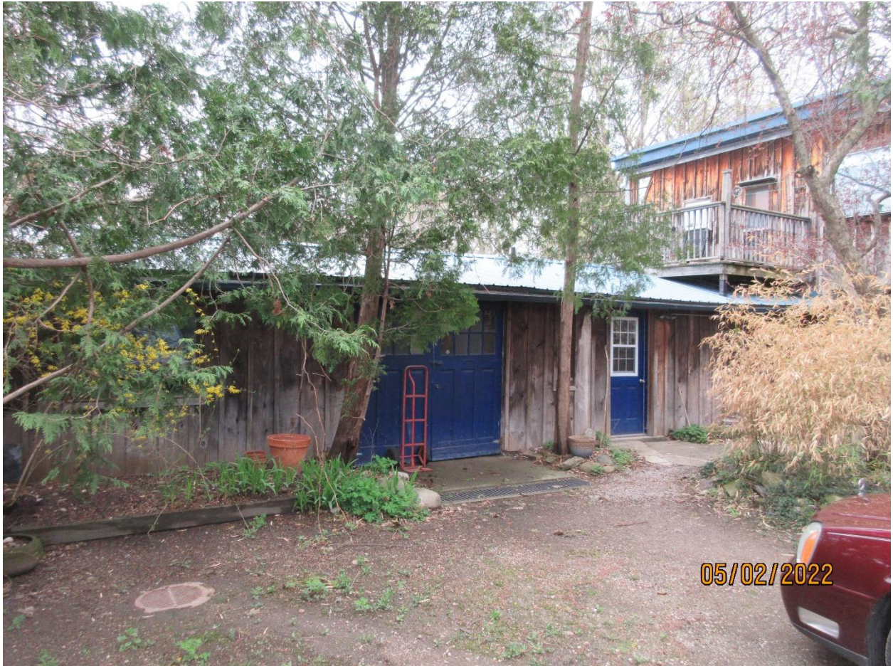
Image 5: View of the garage wing of the building at 514 Pall Mall Street.
