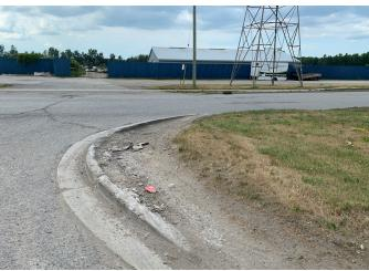
The design at River Road and Scalan Street is much different. The intersection comes to less of a point with more paving present to allow for the large turning radius of the trucks.
