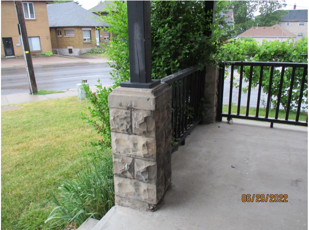
Image 3: Photograph showing porch details on the dwelling at 672 Hamilton Road. Note, the posts and railing system have been replaced.
