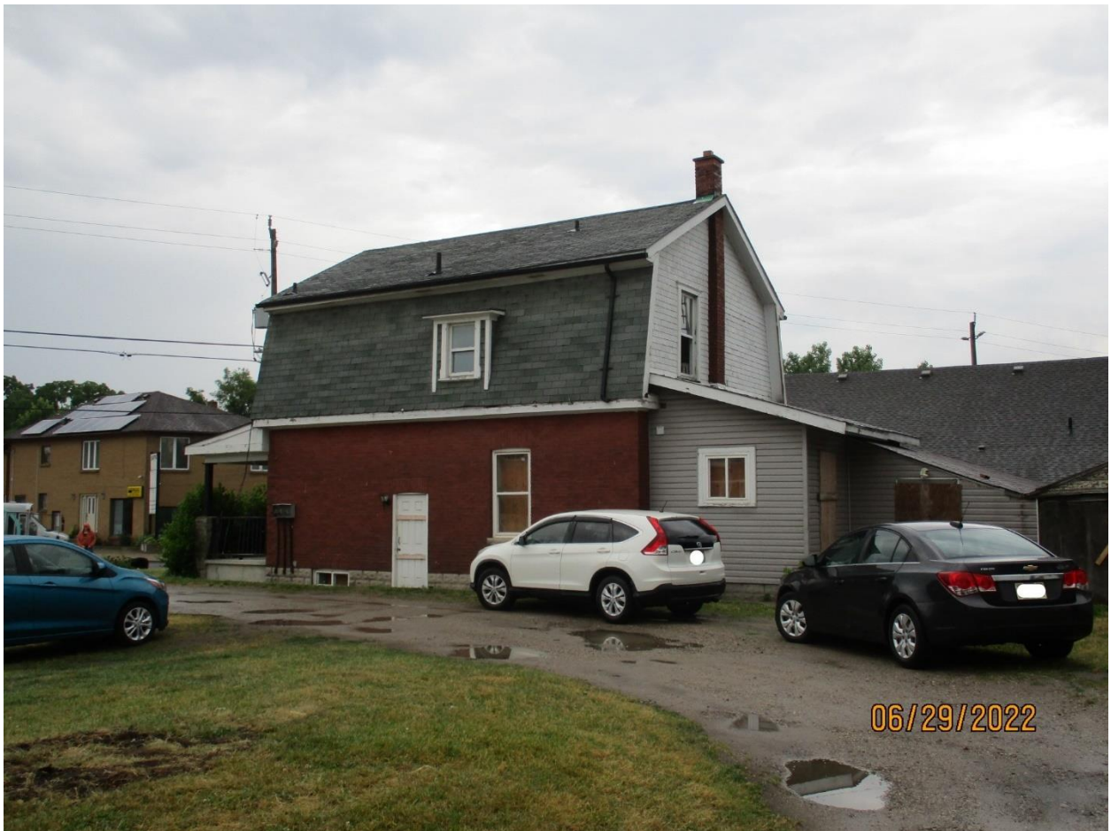
Image 6: Photograph of the sides and rear elevation showing the rear additions.
