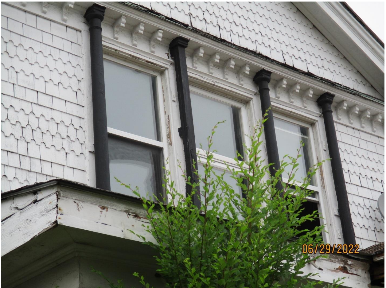
Image 4: Photograph showing detail of the wood columns located between the set of windows on the front elevation of the dwelling. Note, the second column from the left appears to have been replaced.
