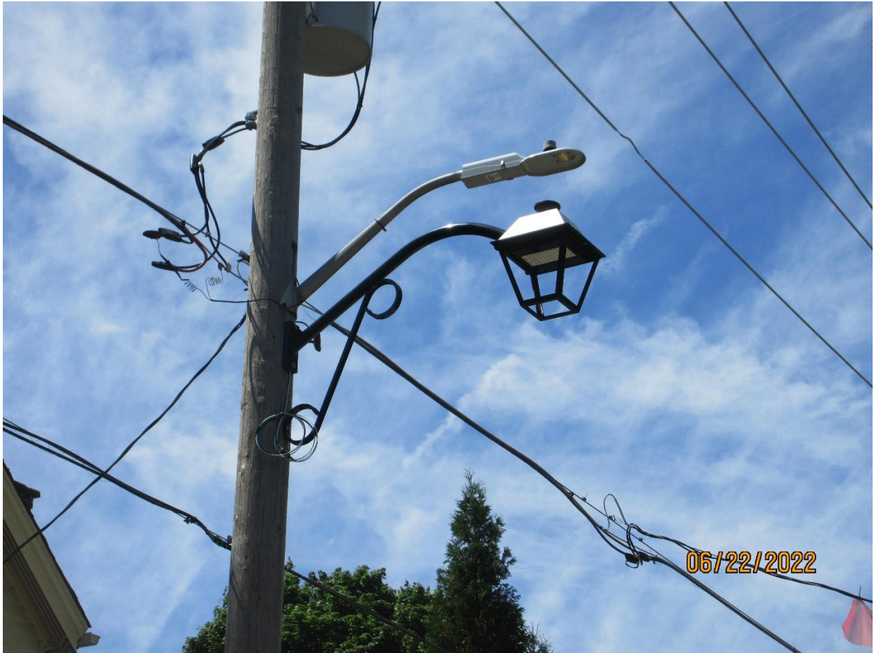
Image 5: Photograph of the new heritage sympathetic light fixture, contrasted to the standard "cobra" light fixtures, being installed on English Street. The "cobra" light fixtures will be removed.
