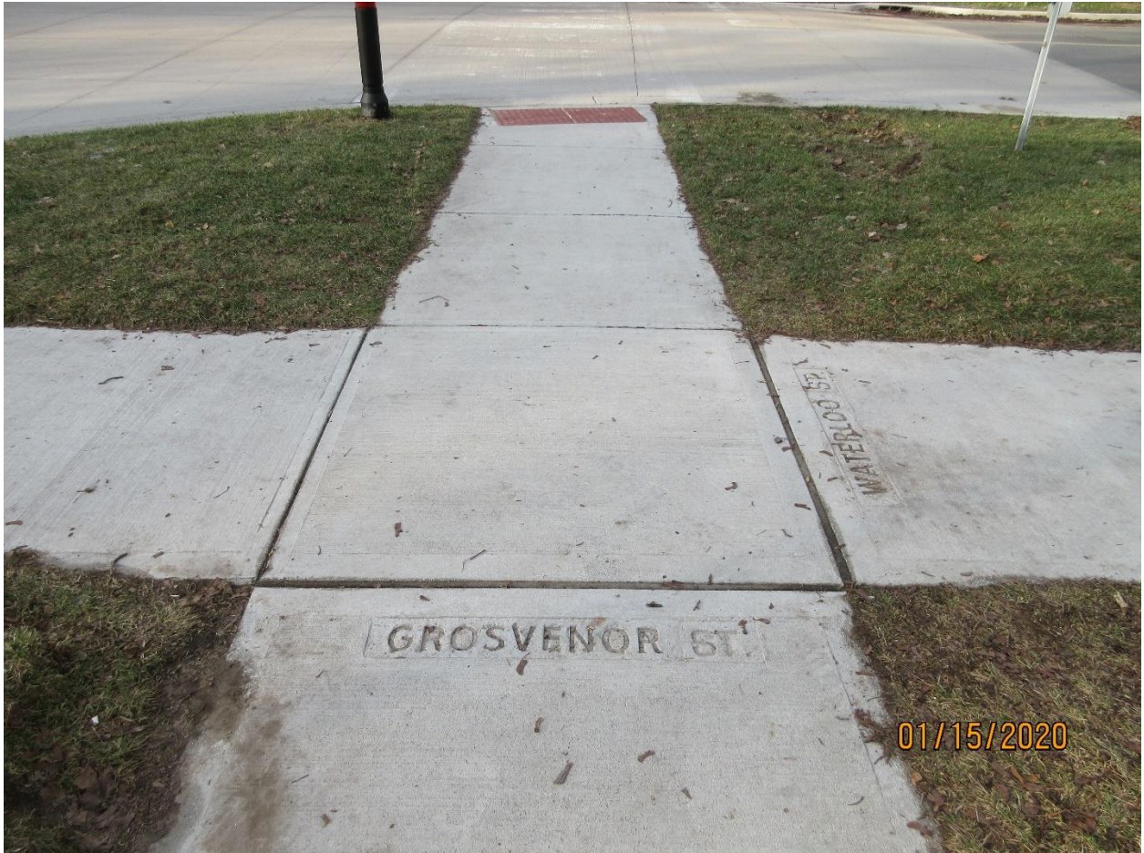
Image 4: Photograph showing the street name stamping, recently completed at Grosvenor Street and Waterloo Street in the Bishop Hellmuth Heritage Conservation District.
