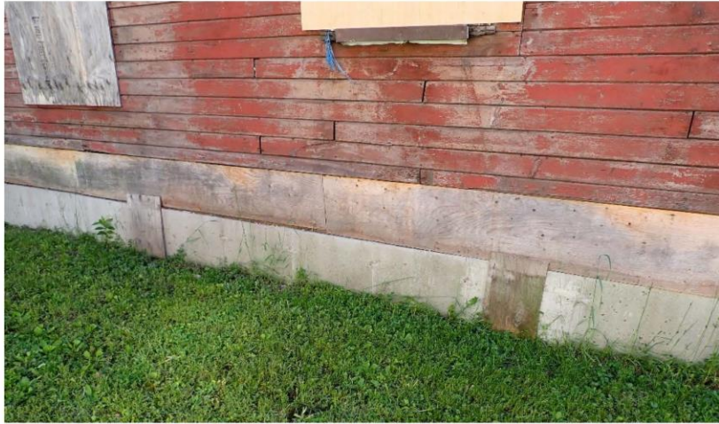
Photographs 3 : Slots in top of foundation wall to install beams for lifting the building.
