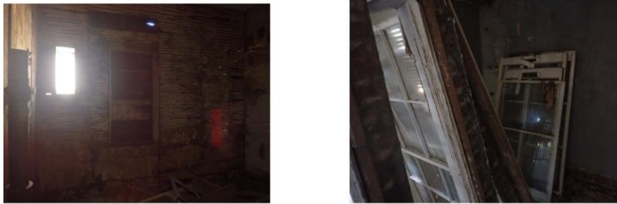
Photographs 8 & 9: North-west and South-West rooms.
