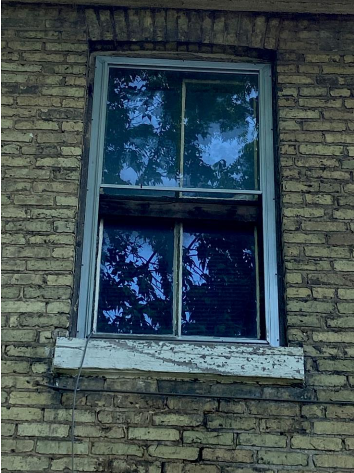
Image 13. Detail of window opening – 2 nd floor, west elevation – showing shallow arch with voussoirs and two-over-two (2/2) wooden window frame and wood sill
