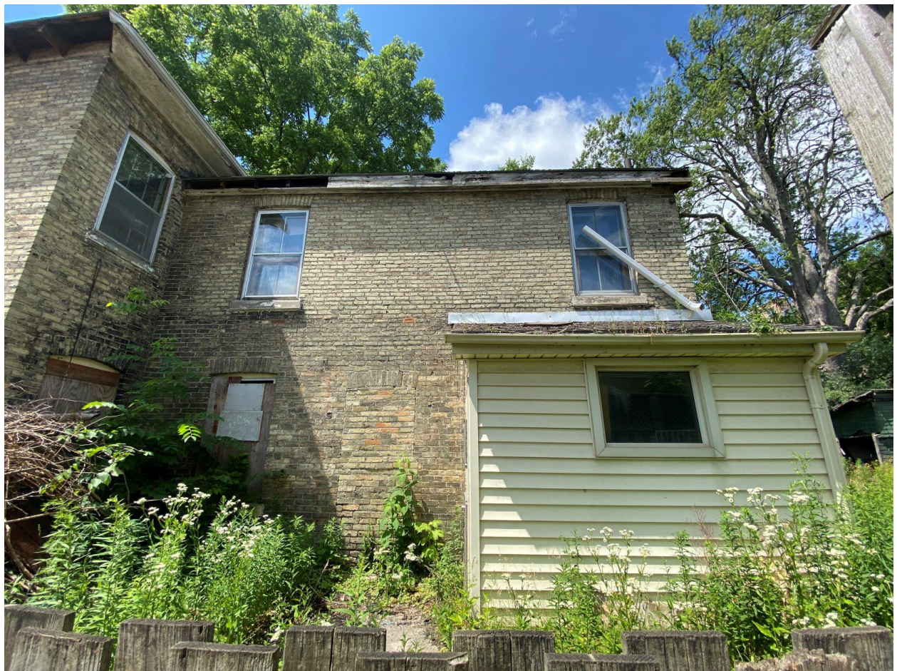
Image 6. East elevation showing rear (north) projection and added entrance vestibule
