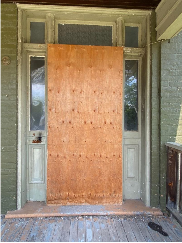
Image 9. Front entrance door surround with transom and sidelites
