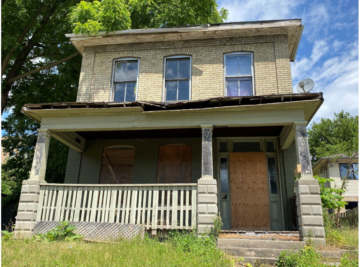
Image 1. Front elevation at 254 Hill Street – facing south
