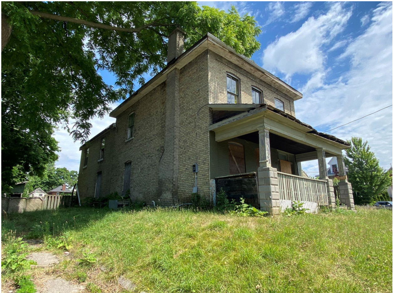
Image 2. South-west elevations at 254 Hill Street
