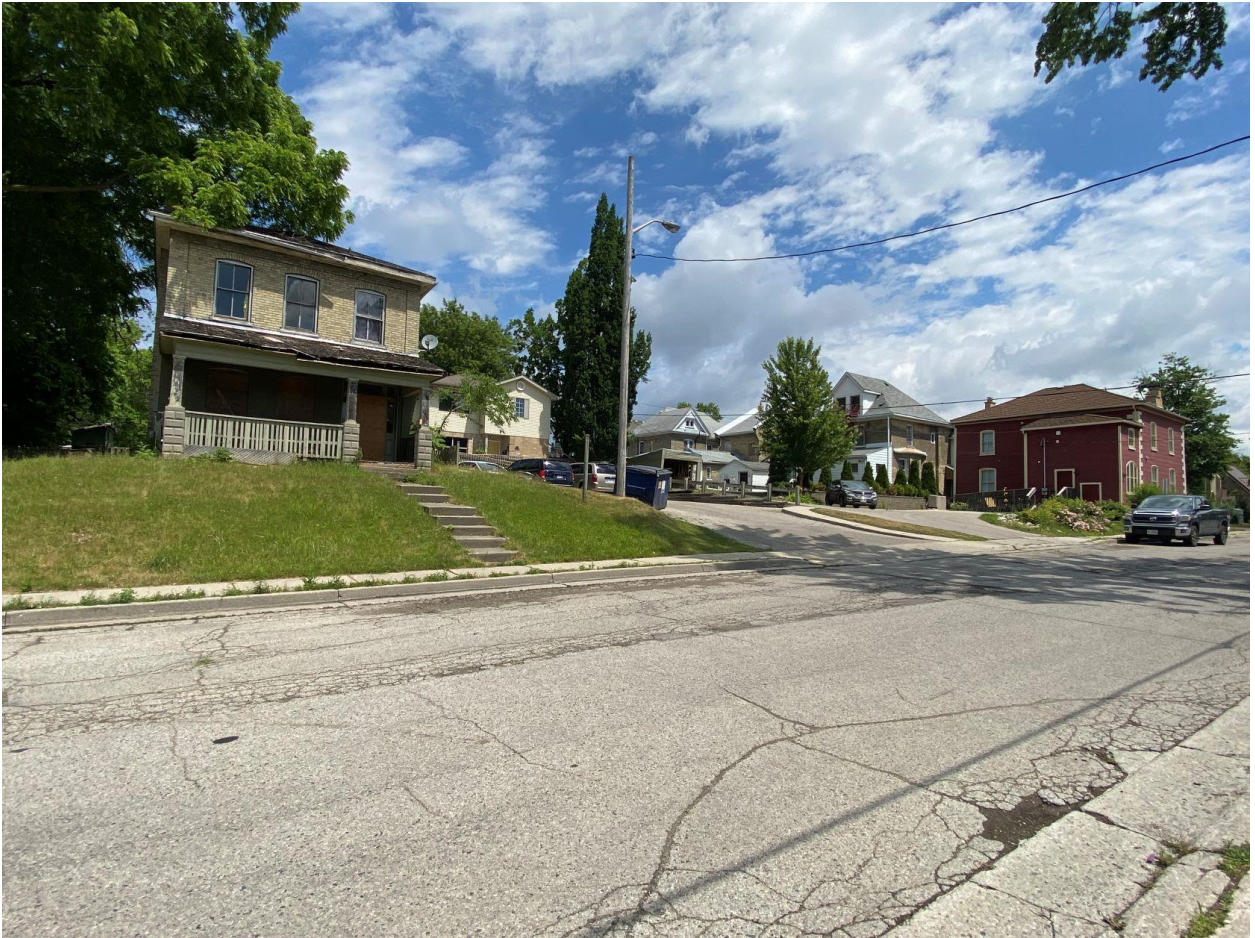
Image 11. Front elevation at 254 Hill Street showing positioning on embankment
