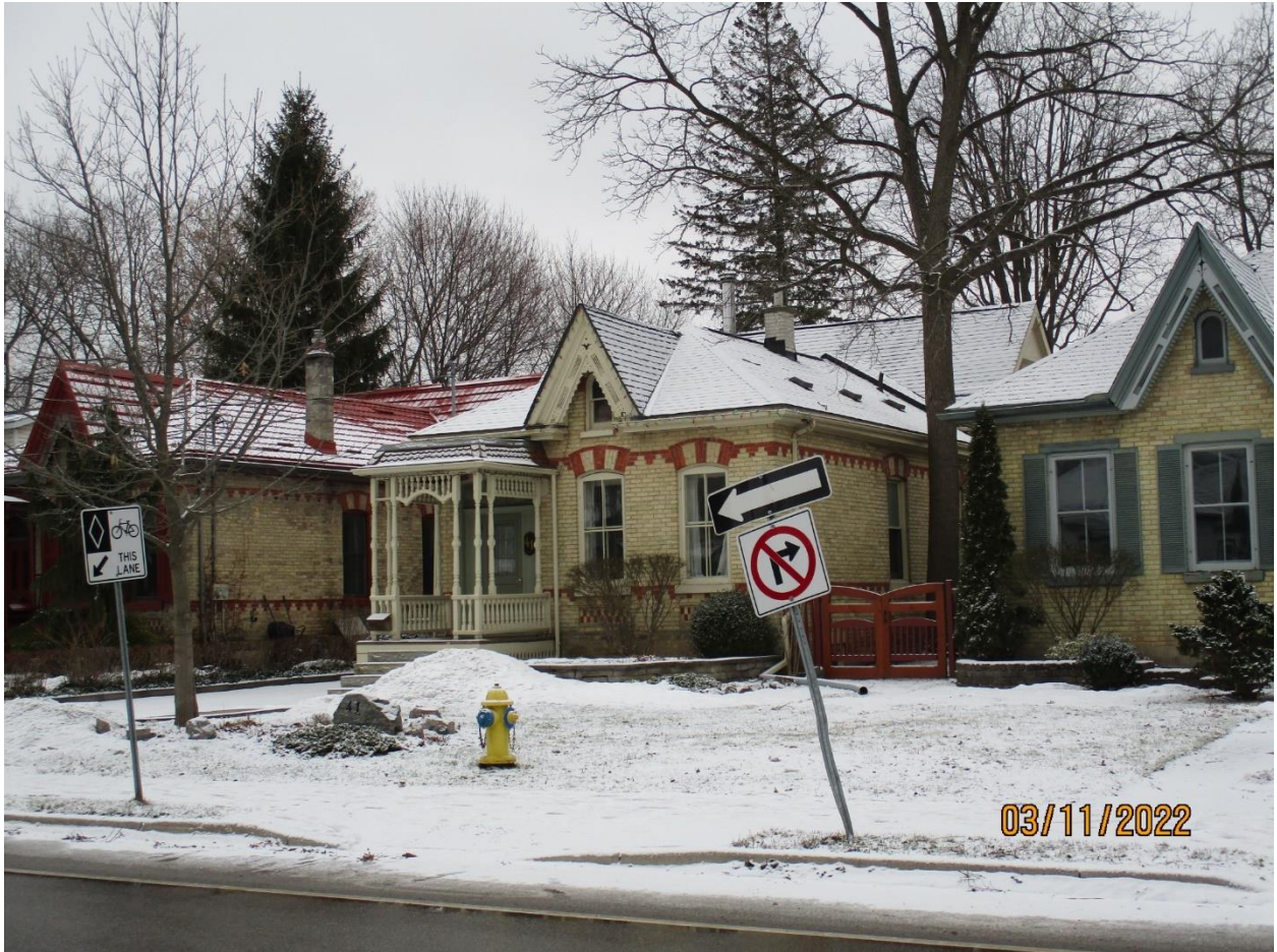
Image 3: Photograph showing 41 Bruce Street (centre) and 43 Bruce Street (left), two of the four nearly identical dwellings on the south side of Bruce Street, located within the Wortley Village-Old South Heritage Conservation District (2022).
