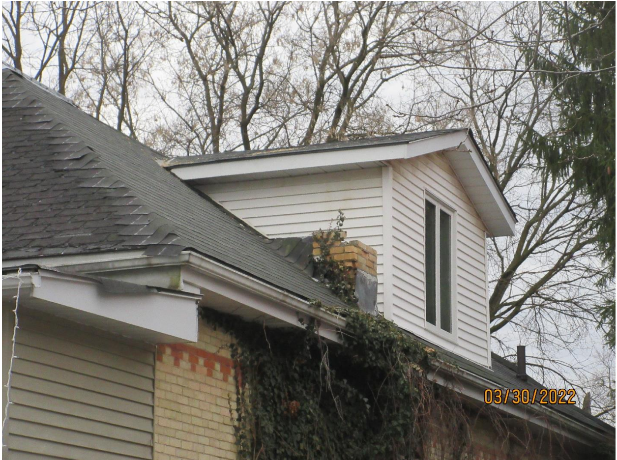
Image 11: Photograph of the chimney following its further removal in March 2022.
