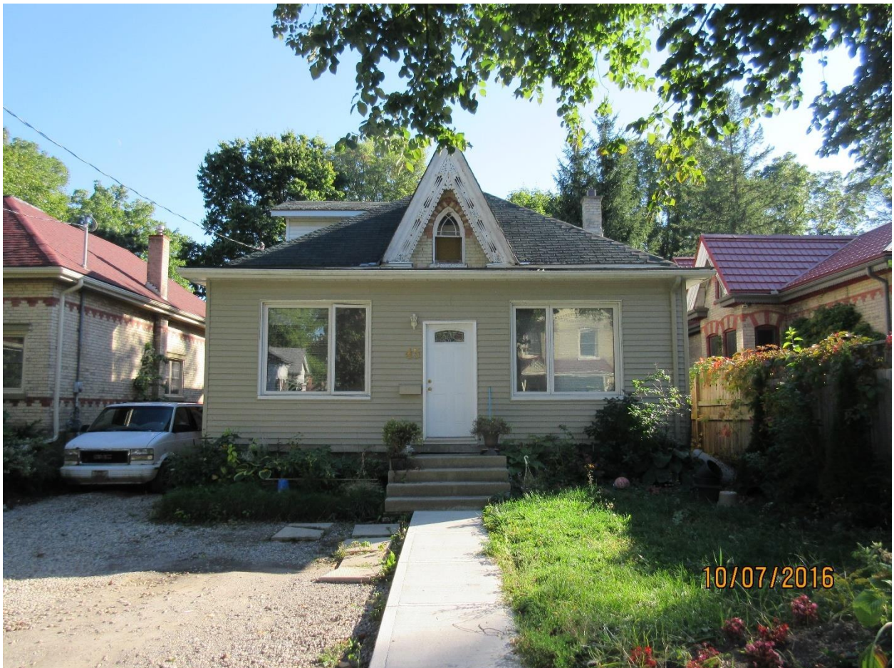
Image 6: Photograph of the subject dwelling at 45 Bruce Street. Note, the front elevation has is obscured by a later addition that has been clad in vinyl, however, the dwelling still retains its cultural heritage value and various heritage attributes, including the scale and mass, and design details including the roof shape, gable peak, brick details visible on side elevations, and brick chimney (2016).
