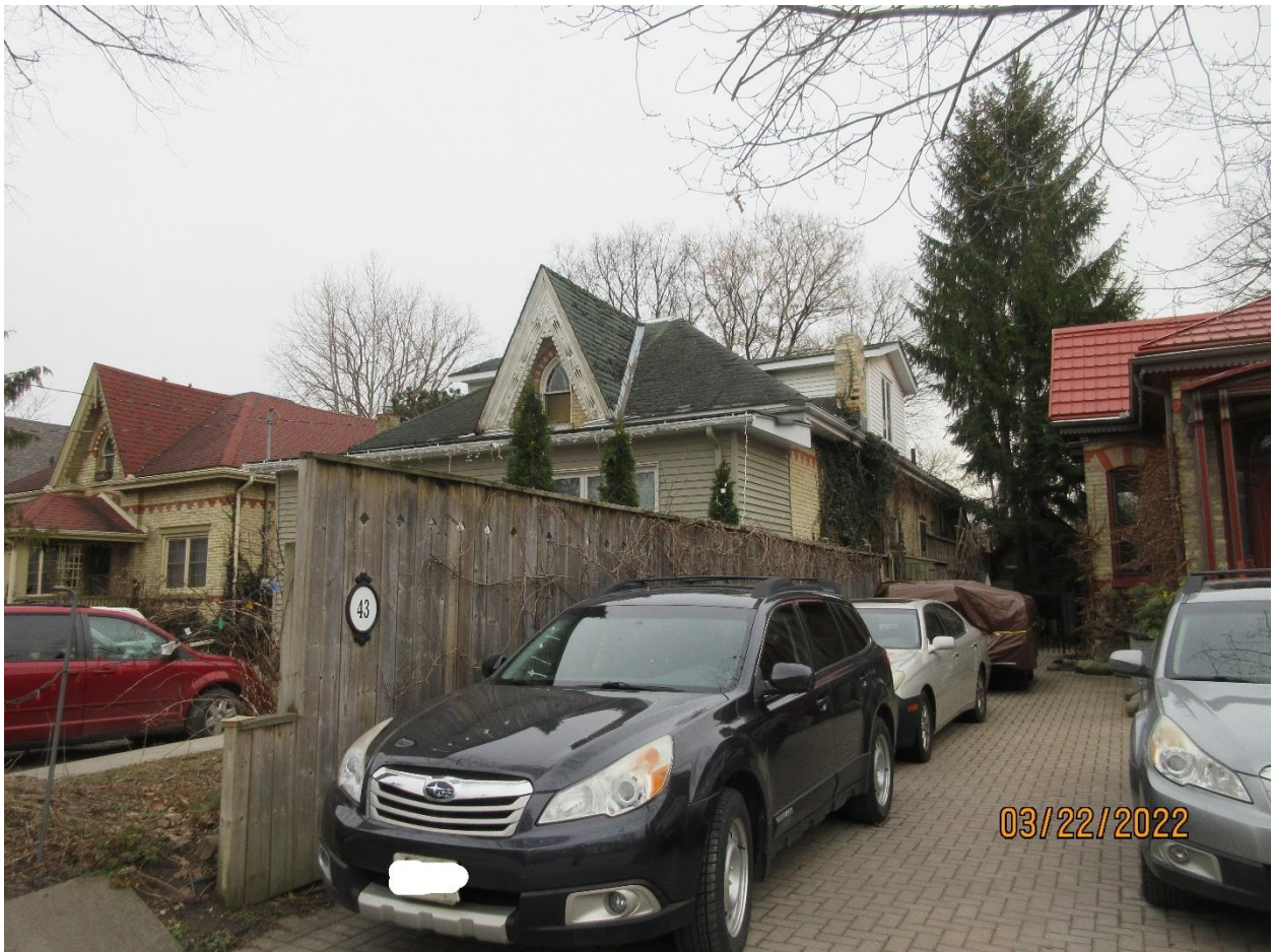
Image 8: Photograph of the subject dwelling at 45 Bruce Street, shortly after the partial collapse of the chimney. Note, the decorative dichromatic brick on the side elevations of the dwelling can be observed in this photograph as well as on the adjacent properties (2022).
