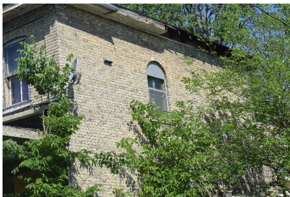
Plate 23: Arched window of east elevation, looking northwest
