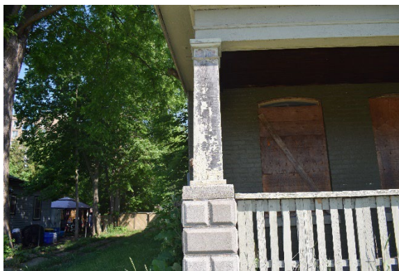
Plate 15: Close-up of concrete block and wood columns of porch
