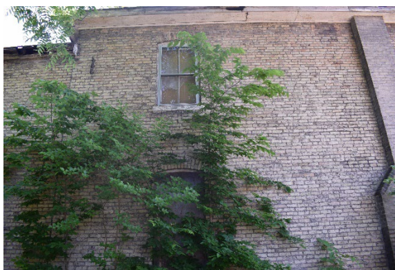
Plate 17: Windows of the principal section of the west elevation
