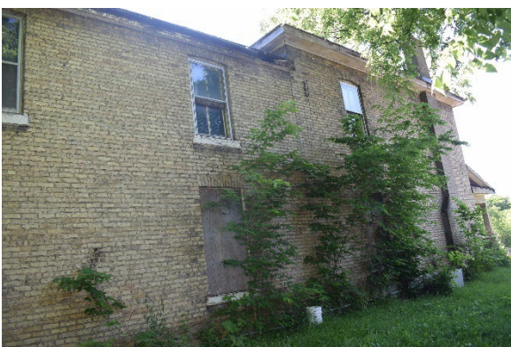
Plate 16: Looking southeast at the two sections of the west elevation
