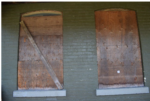
Plate 13: Boarded windows, looking north elevation
