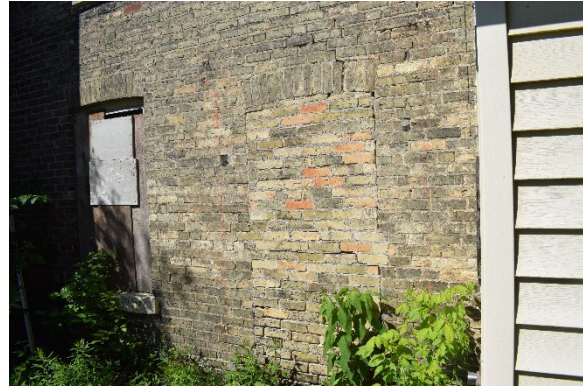
Plate 25: Boarded window and bricked over doorway, looking west
