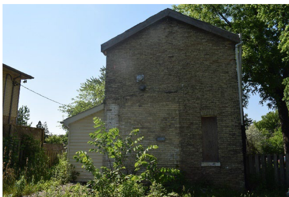
Plate 19: North elevation of gable projection, looking south
