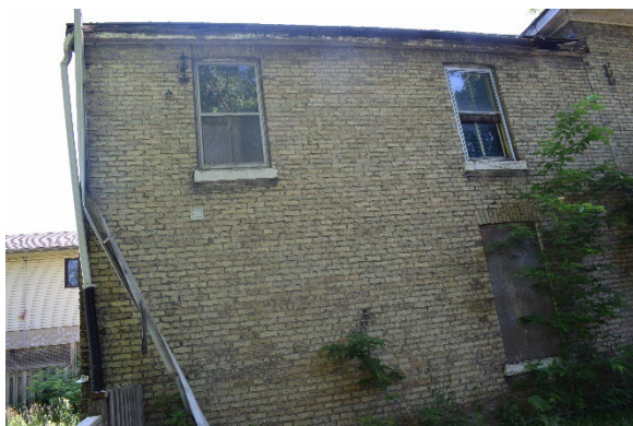
Plate 18: Windows of the gable roof projection, looking east
