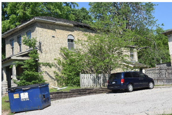
Plate 22: Looking west at east elevation
