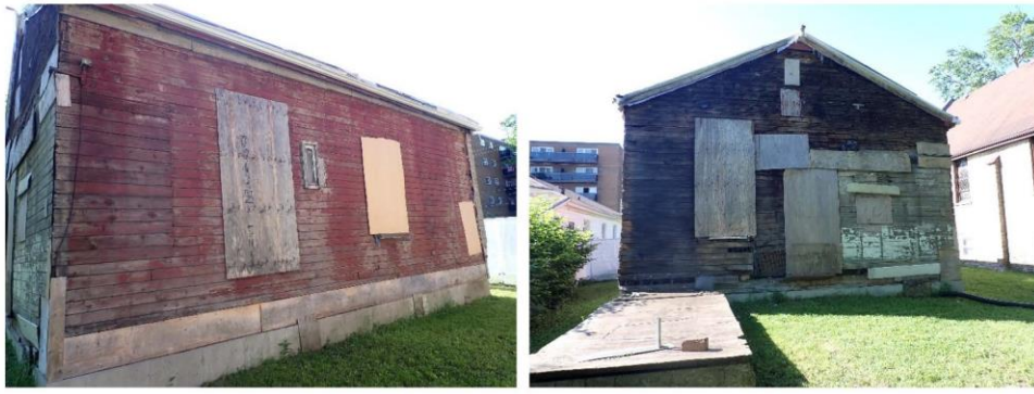
Photographs 4 & 5: West and North Elevations
