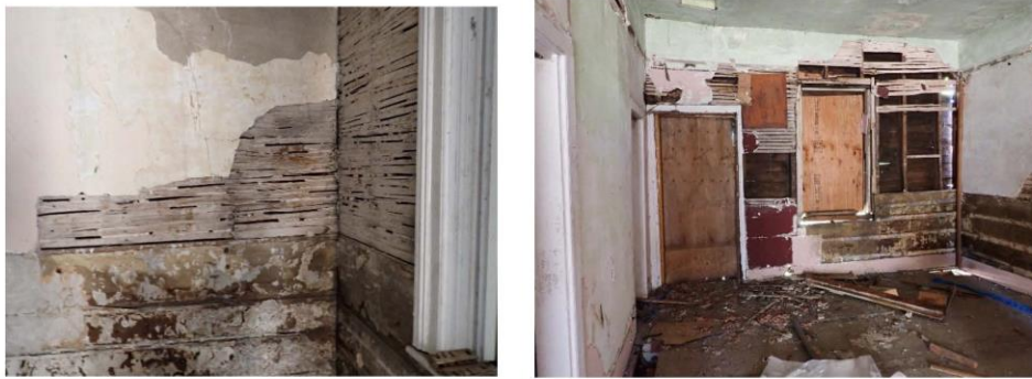
Photographs 6 & 7: Interior wood lathe and plaster wall sheathing. Main room (east side)
