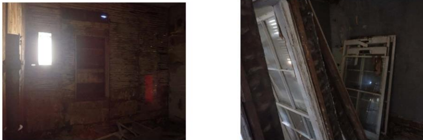
Photographs 8 & 9: North-west and South-West rooms.
