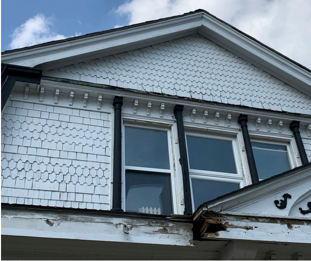
Photo #9: Details typical of the Dutch Colonial Revival Style:
