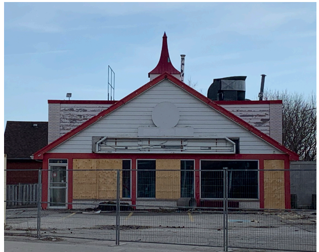
Photo #8: 689 Hamilton Road. Built in 1947. City of London: Register of Cultural Heritage Resources, July 2, 2019. Source: City of London.
