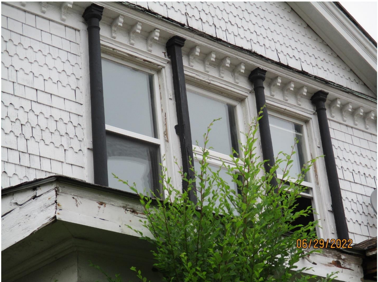
Image 4: Photograph showing detail of the wood columns located between the set of windows on the front elevation of the dwelling. Note, the second column from the left appears to have been replaced.
