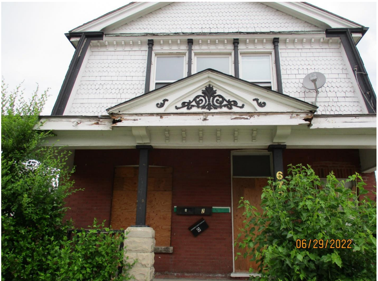
Image 2: Photograph showing porch details on the subject dwelling at 672 Hamilton Road.
