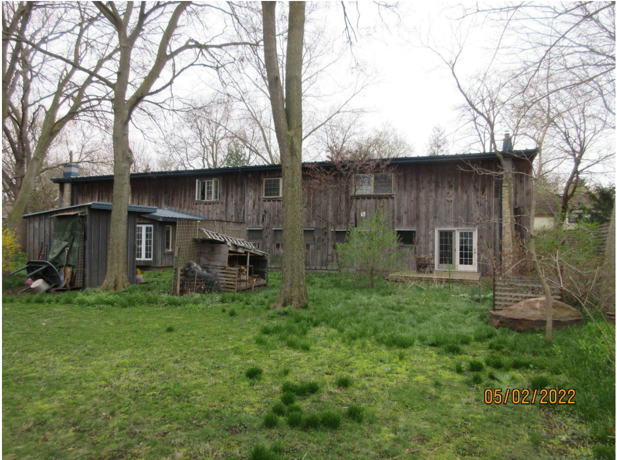
Image 3: View of the east façade of the building at 514 Pall Mall Street.
