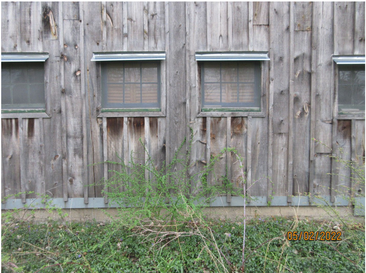
Image 4: Detail of four of the horse stall windows on the east façade of the building at 514 Pall Mall Street. There are fourteen horse stall windows on the building, articulating its origins as a stable.
