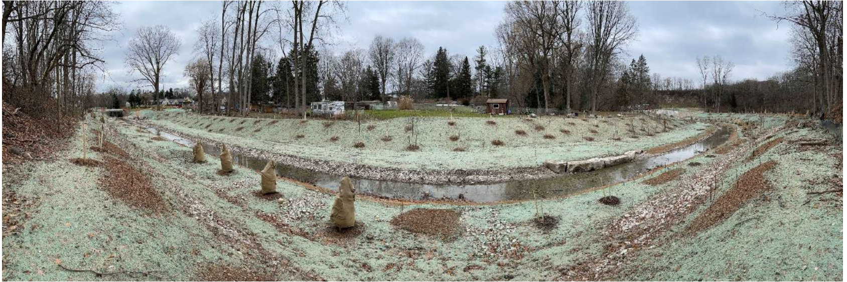
Mud Creek Rehabilitation (Phase 1 - 2021)
